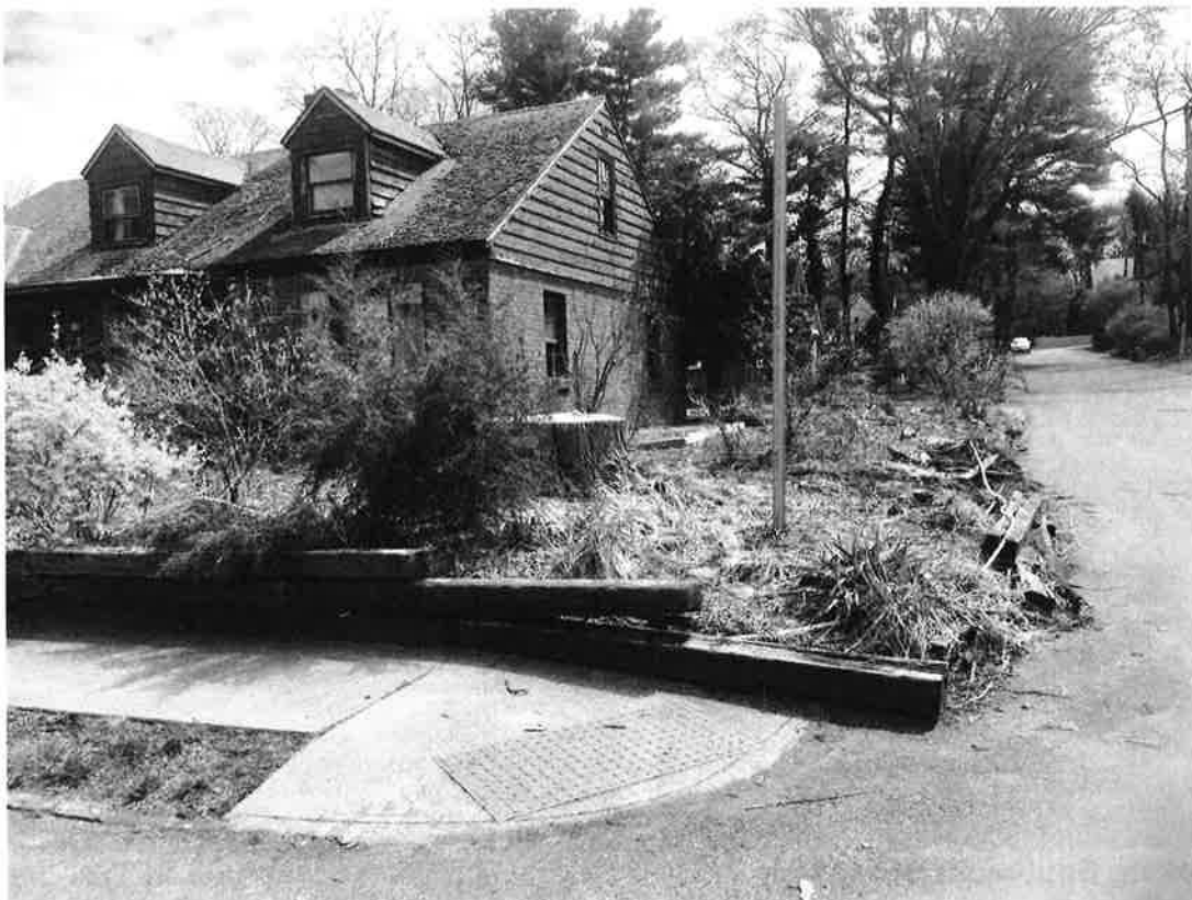
Corner and side yard encroachment into Sharon Street right of way
