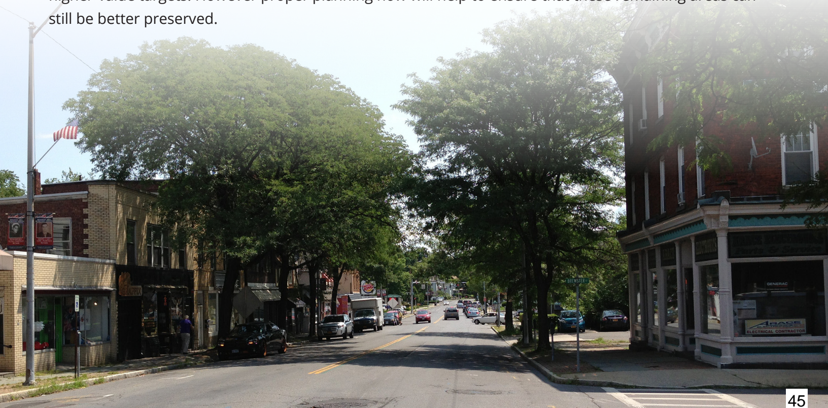
Figure 6. The intersection of Broadway and Brewster Street.
