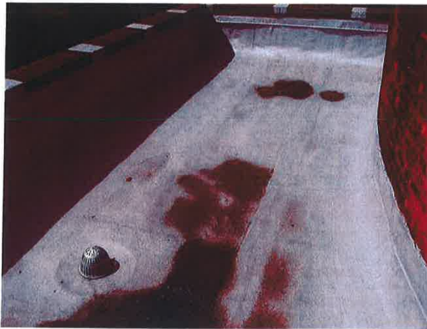
Heat Exchange Room, Newer Roof over BUR
