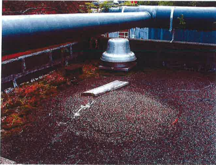
Primary Building Roof and Flashings
