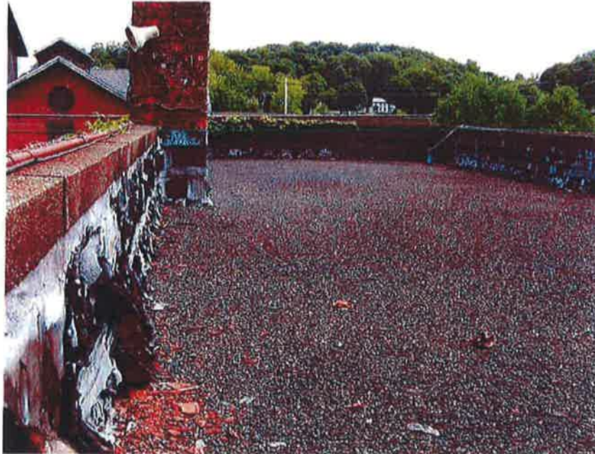
Primary Building Roof and Flashings
