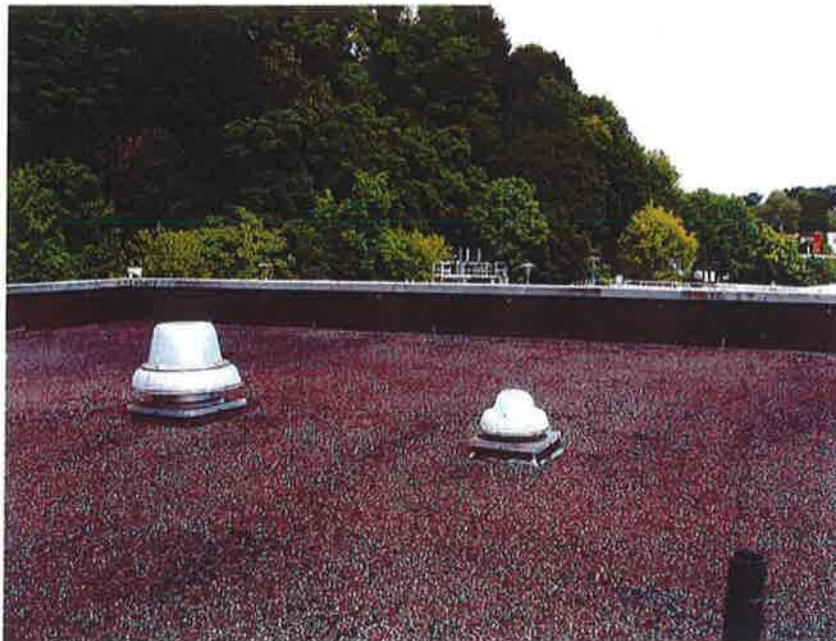
Main Control Building Mid Level Roof, Flashing and Coping
