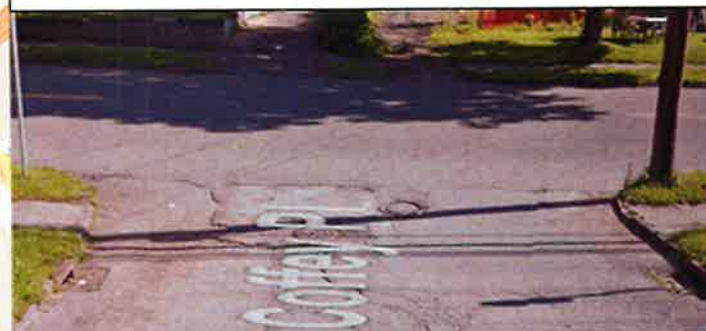
Photo: curb ramps at the intersection of Hurley Ave and Coffey Pl
