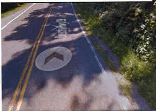
Photo: view of existing shoulder on Hurley Ave, facing the Thruway
