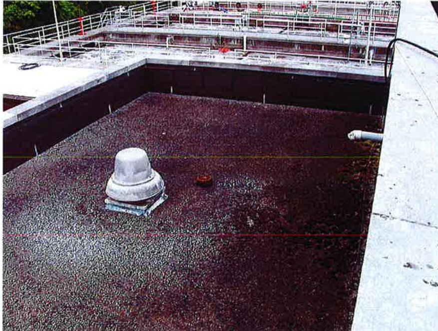
Main Control Building Lower Roof, Flashing and Coping
