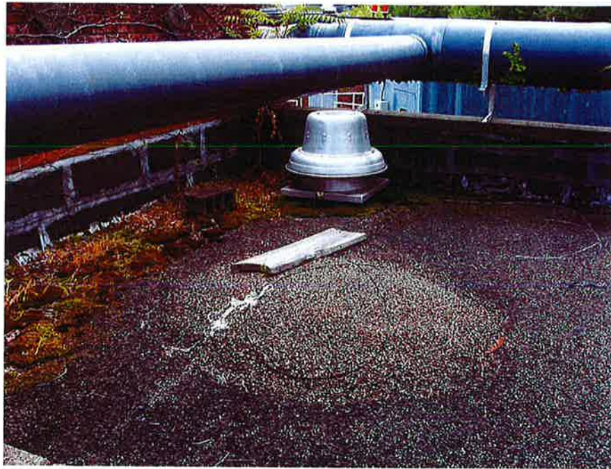
Primary Building Roof and Flashings
