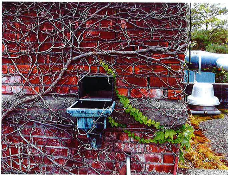
Primary Building Roof: Thru-Wall Scupper
