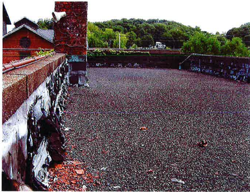
Primary Building Roof and Flashings
