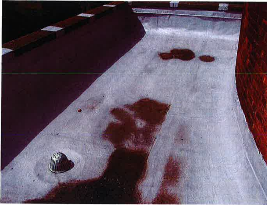
Heat Exchange Room, Newer Roof over BUR
