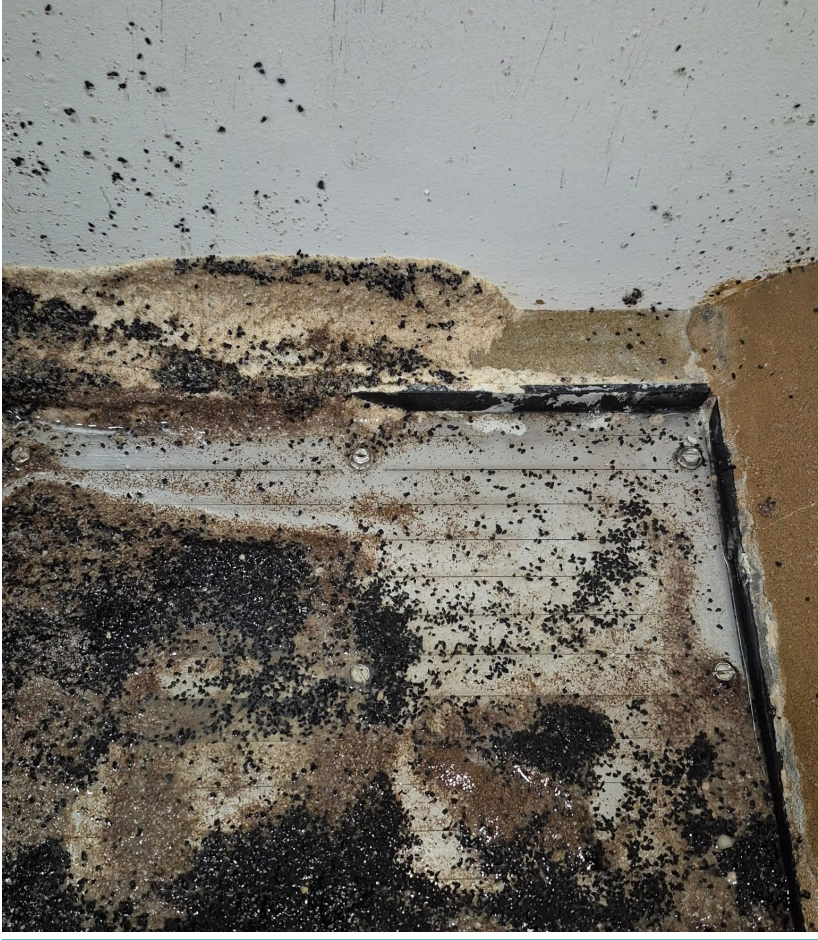
Observed panel and grout area.
