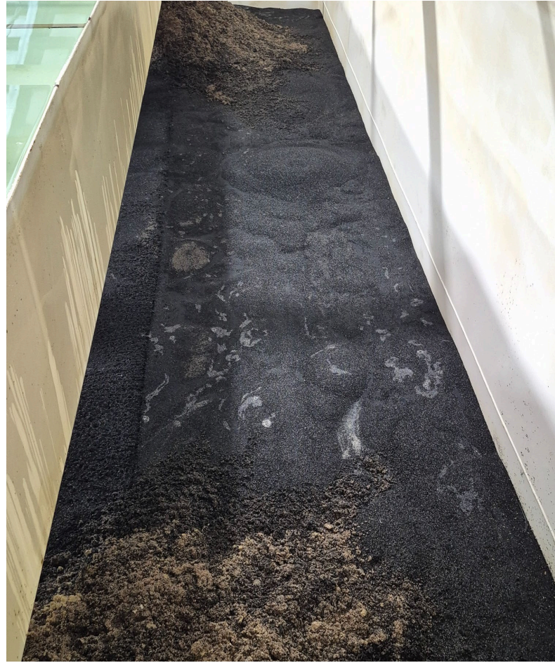
Trident Unit drained and Filter media dug out in three locations.
