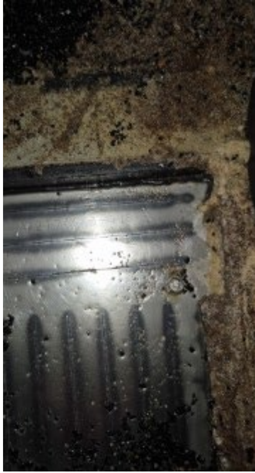
Close-up of observed condition.
