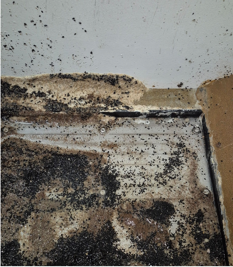
Observed panel and grout area.
