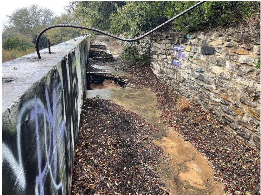
Figure 07. Holes in flatwork behind lower wall, due to soil cave-in
