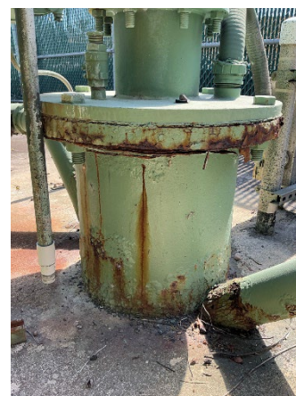
Raw Water Well No. 10
