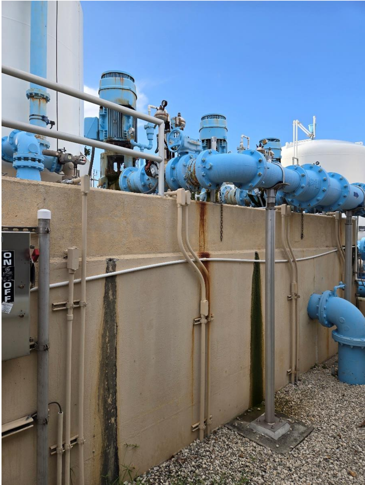
Front of Clearwell
