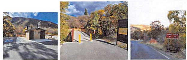
FOREBAY — EASE OF ACCESSIBILITY
