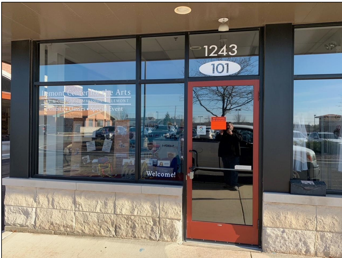
Figure 4: Not approved for occupancy notice.
