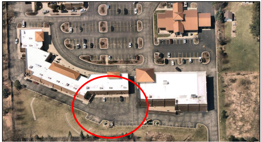
Figure 1: Approximately 20 parking stalls behind Suite 101.
