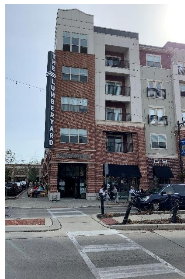
Example of Blade Sign, Collingswood, NJ
