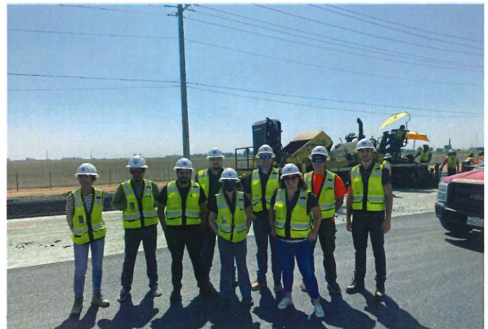
The UNICO team on-site during paving operations at the Kammerer Road Reconstruction project for the City of Elk Grove
