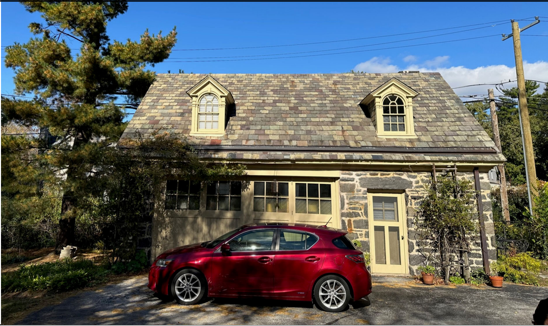
Existing Carriage House
