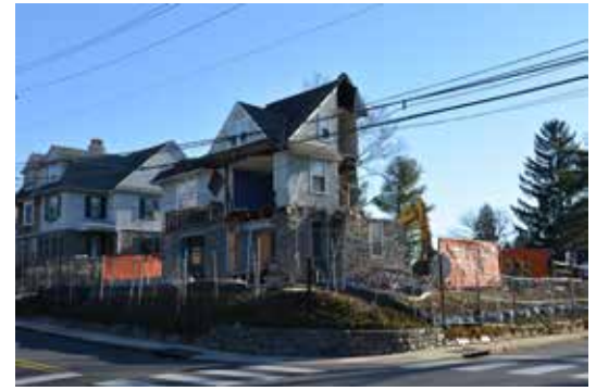
4.17. Instead of being demolished via conventional means like this undesignated early 1900s home in Bryn Mawr, buildings could be deconstructed to preserve valuable materials and decrease the environmental impact of putting reusable building materials in landfills.
