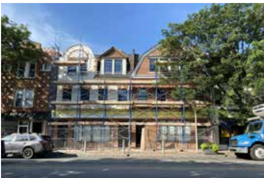
5.8-5.10. The reconstruction of two historic “Colonial Block” façades in downtown Ardmore did not follow the approved plans in terms of proportions, window placement, cornices, and other details. HARB sought to ensure that the work matched the original façade (top) as closely as possible. Work could not be adequately observed while scaffolding was tarped (center), and was only revealed to be out of keeping with the approved plans once tarps were removed (bottom).
