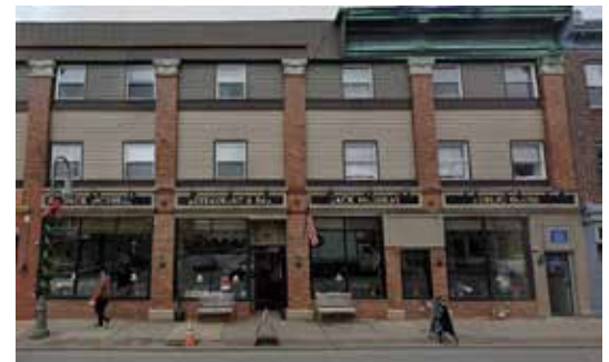
2.25-2.27. Case Study 4: 34 East Lancaster Avenue
