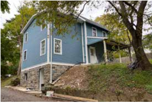
5.11. Smith Cottage during renovations.
