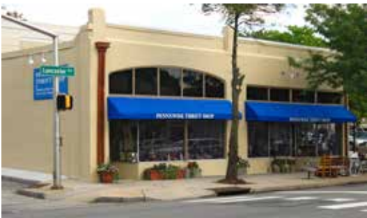
2.12-2.24. Case Study 3: 57-59 East Lancaster Avenue
