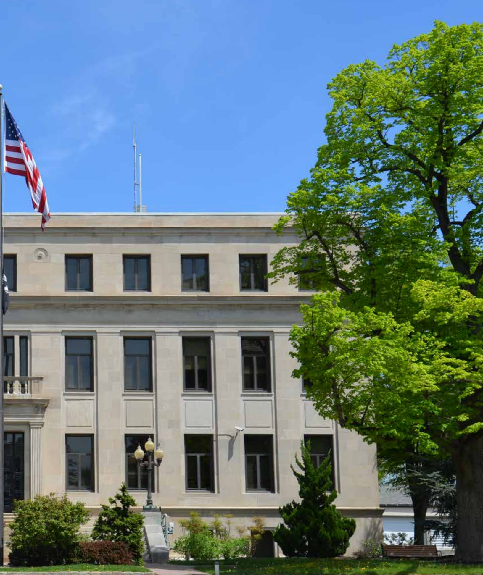
Lower Merion Township Administration Building, Ardmore
