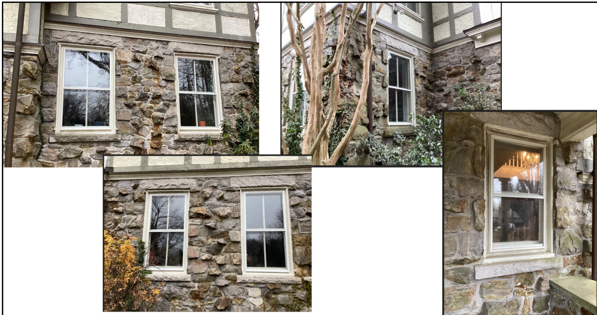
Views of Existing Windows to be Replaced
