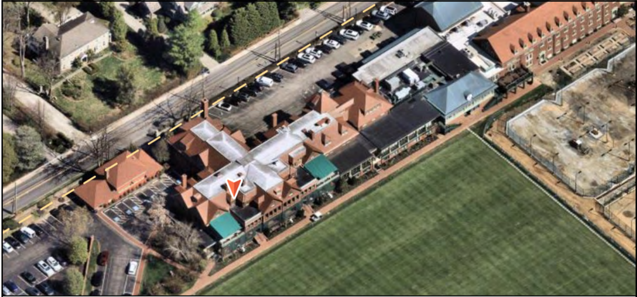
325 Montgomery Avenue, Haverford - Merion Cricket Club
