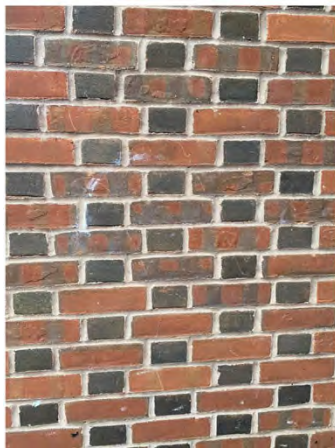
FLEMISH BOND PATTERNED BRICKWORK TO MATCH EXISTING
