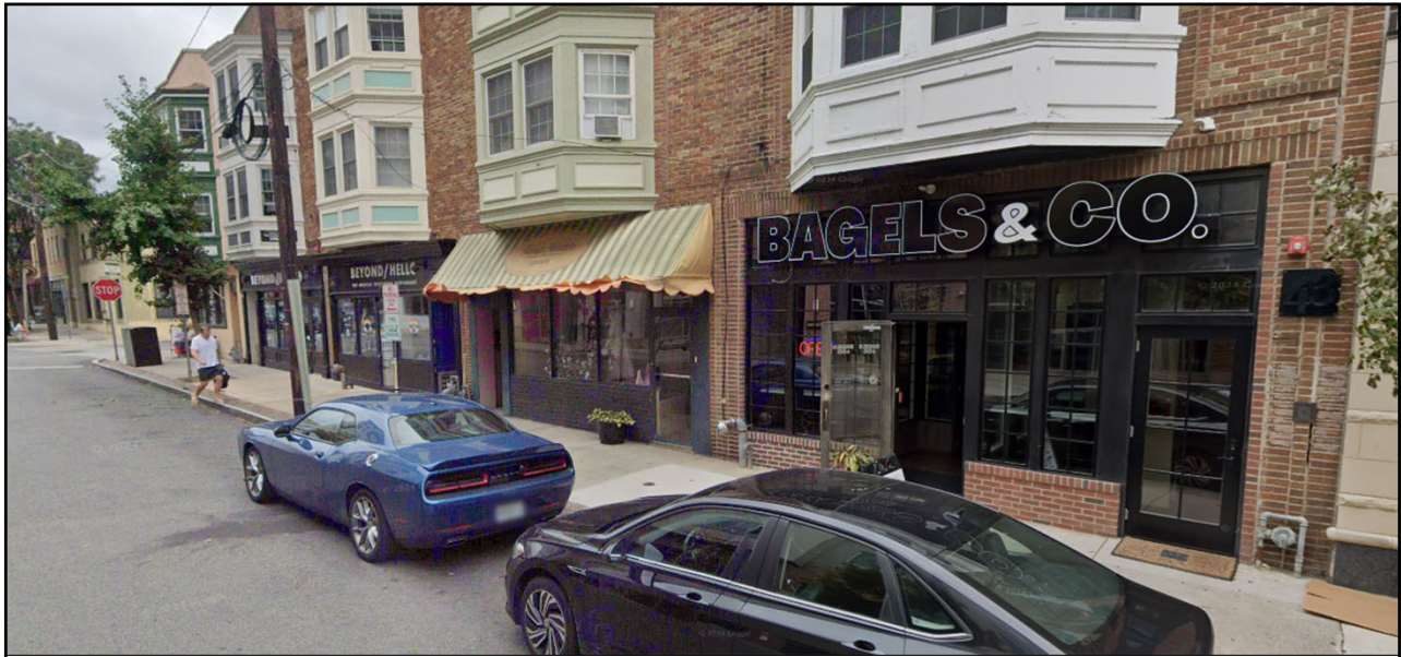
43 Cricket Avenue, Ardmore Commercial Historic District
