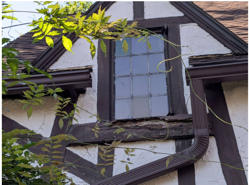
Examples of rotted trim and sills in need of replacement
