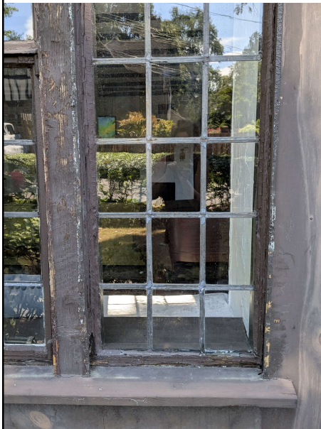
Examples of rotted trim and sills in need of replacement
