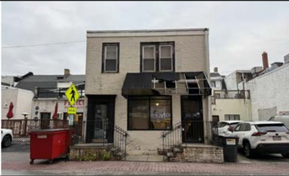
16 West Lancaster Avenue (Rear) – Ardmore Commercial Center Historic District
