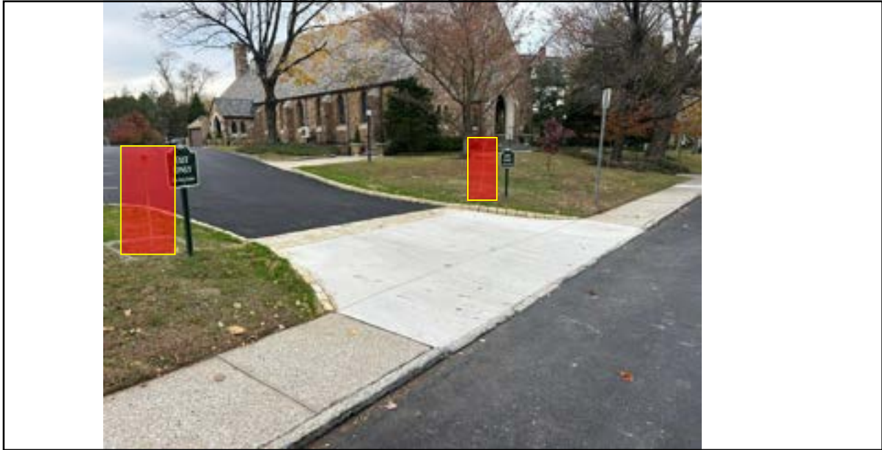
Youngs Ford Road Entrance (Approx. Locations of Piers Highlighted)
