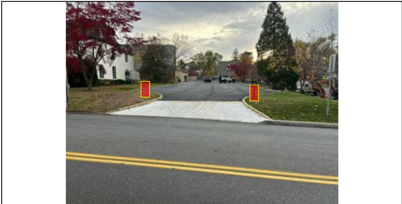
Consh. State Road Entrance (Approx. Locations of Piers Highlighted)
