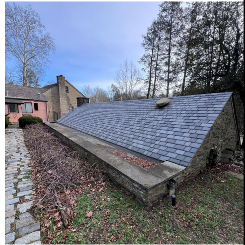
Rear Roof Slope
