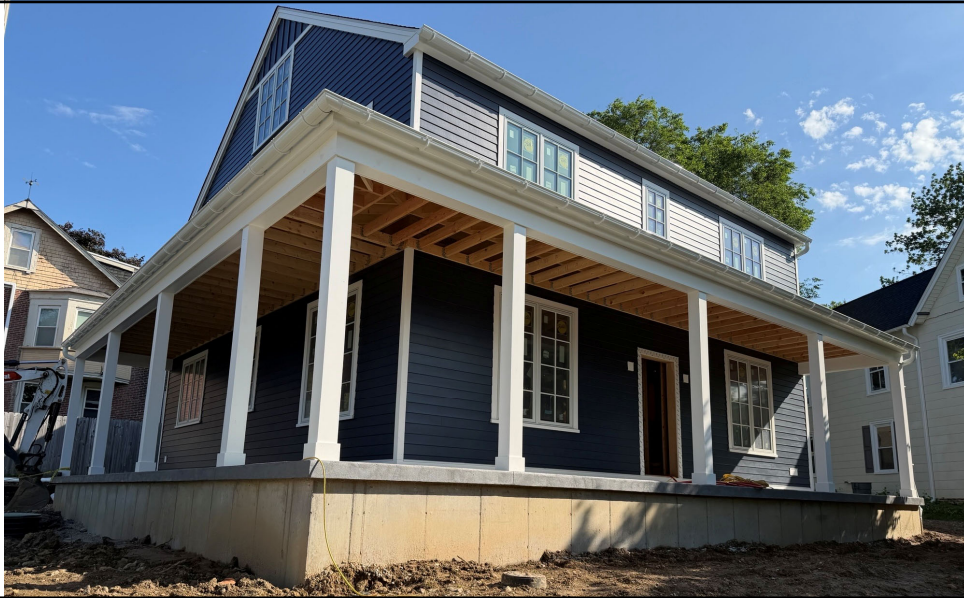
527 Old Lancaster Road – Haverford Station Historic District
