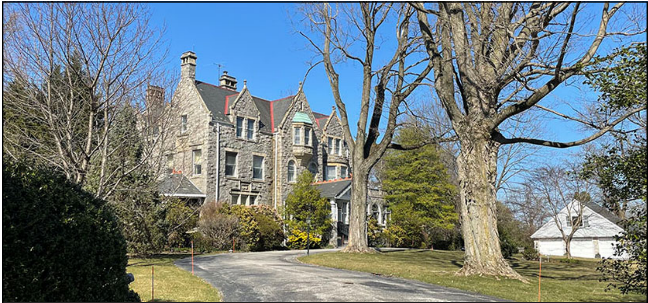
220 Cuylers Lane, Haverford
