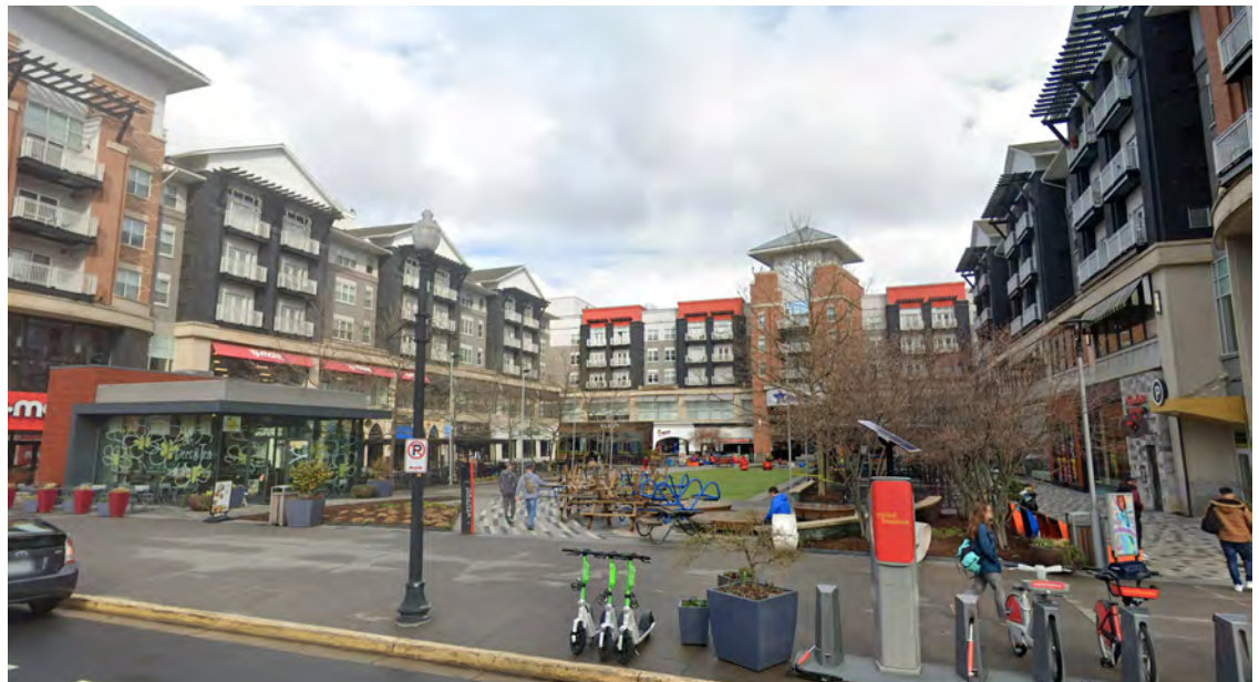
Westpost at National Landing Retail Cluster, Arlington County, VA
