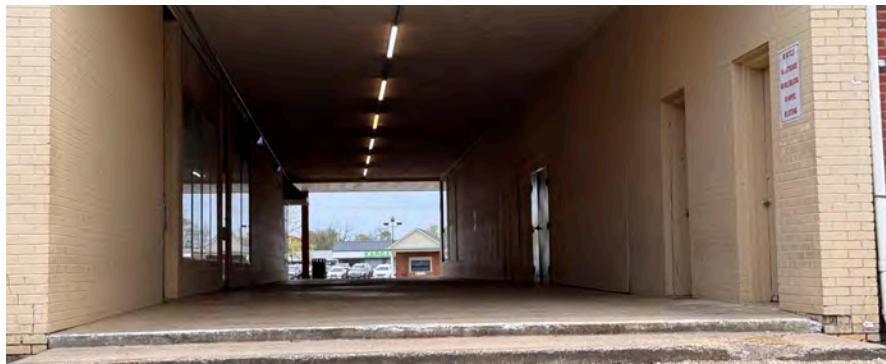
5 Existing breezeway between front and rear of Shopping Center
