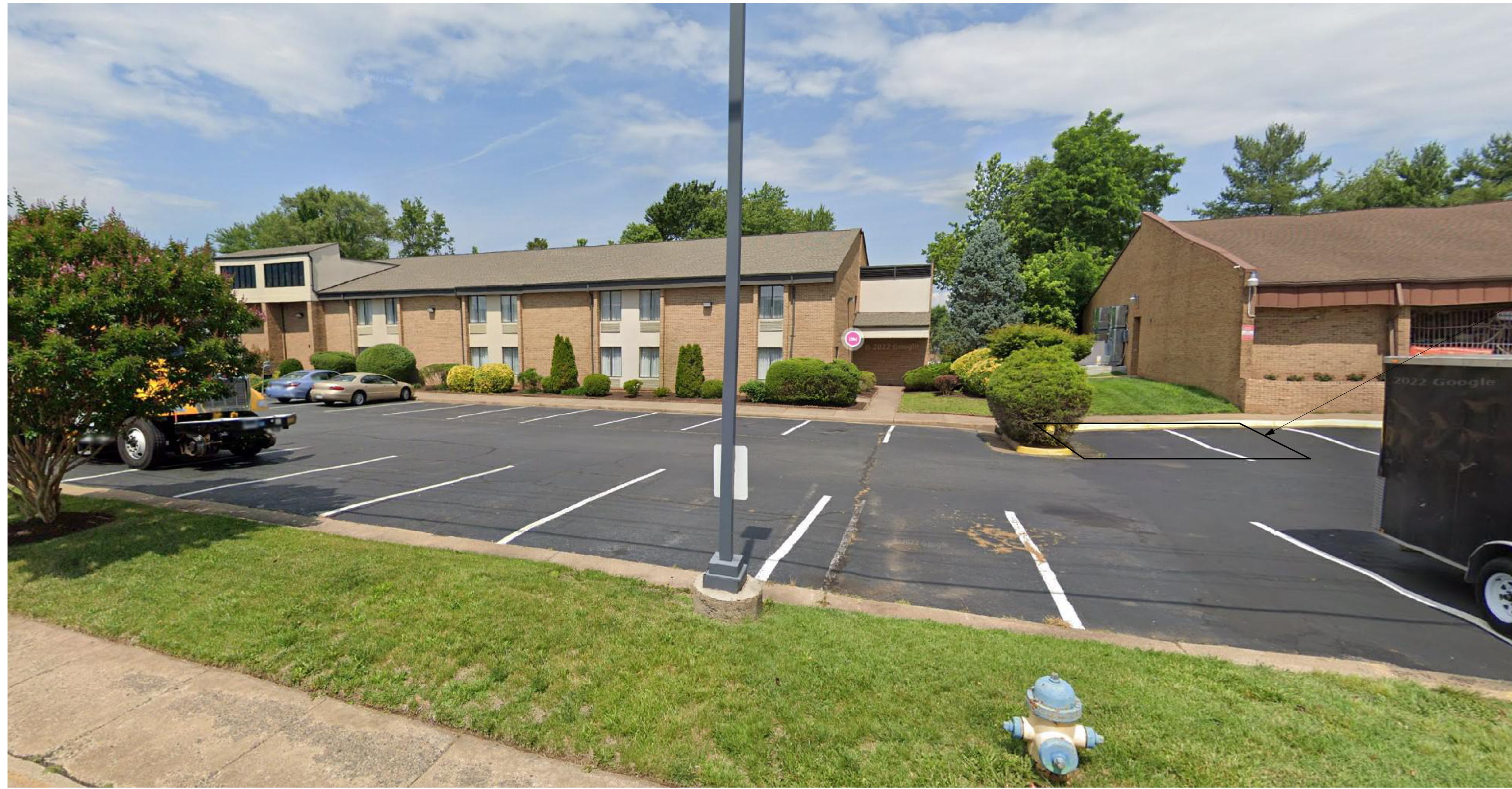
APPROX. DUMPSTER LOCATION
