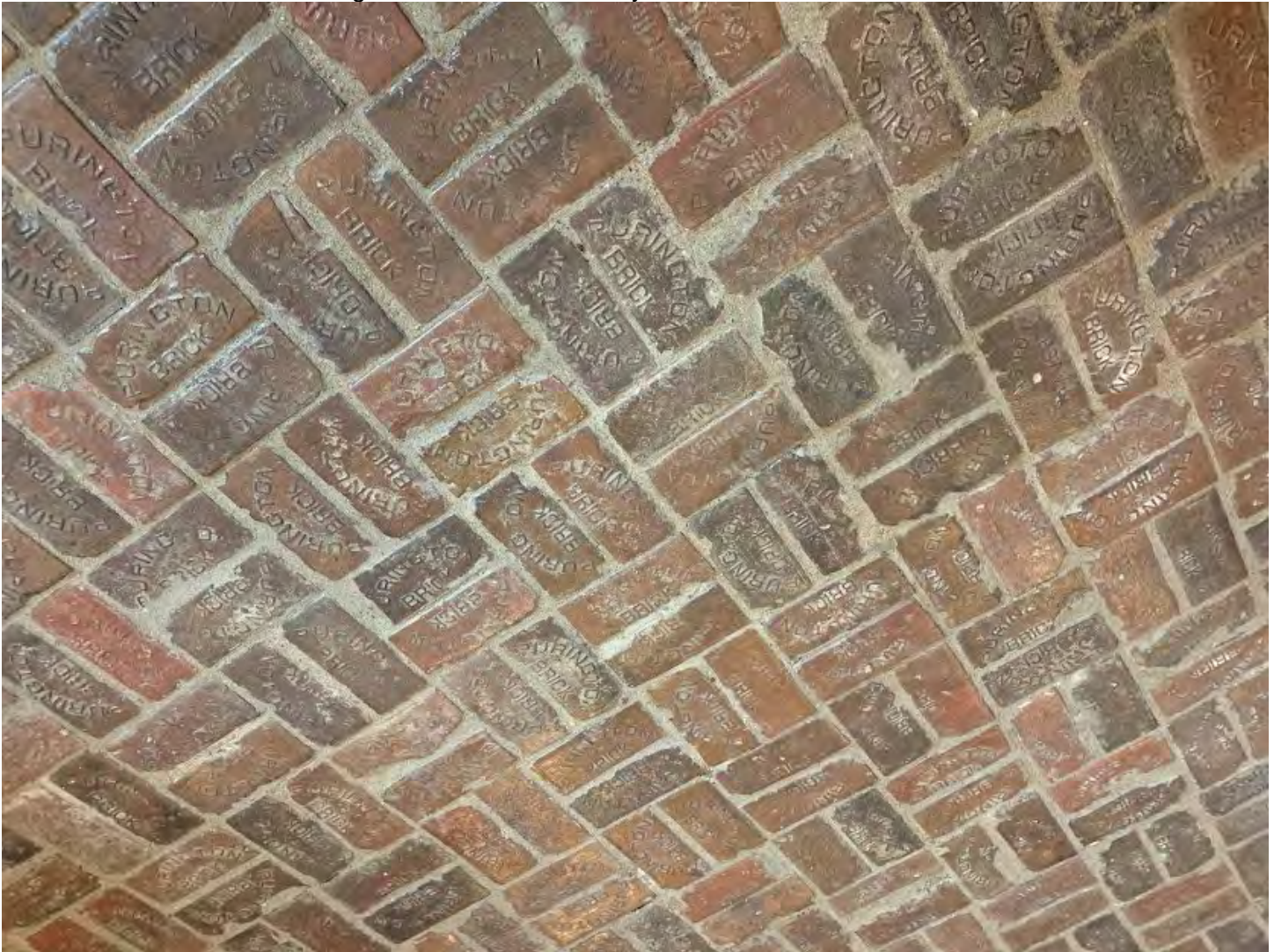
Photo 9 of 11: Restored Purington Bricks in service bay.
