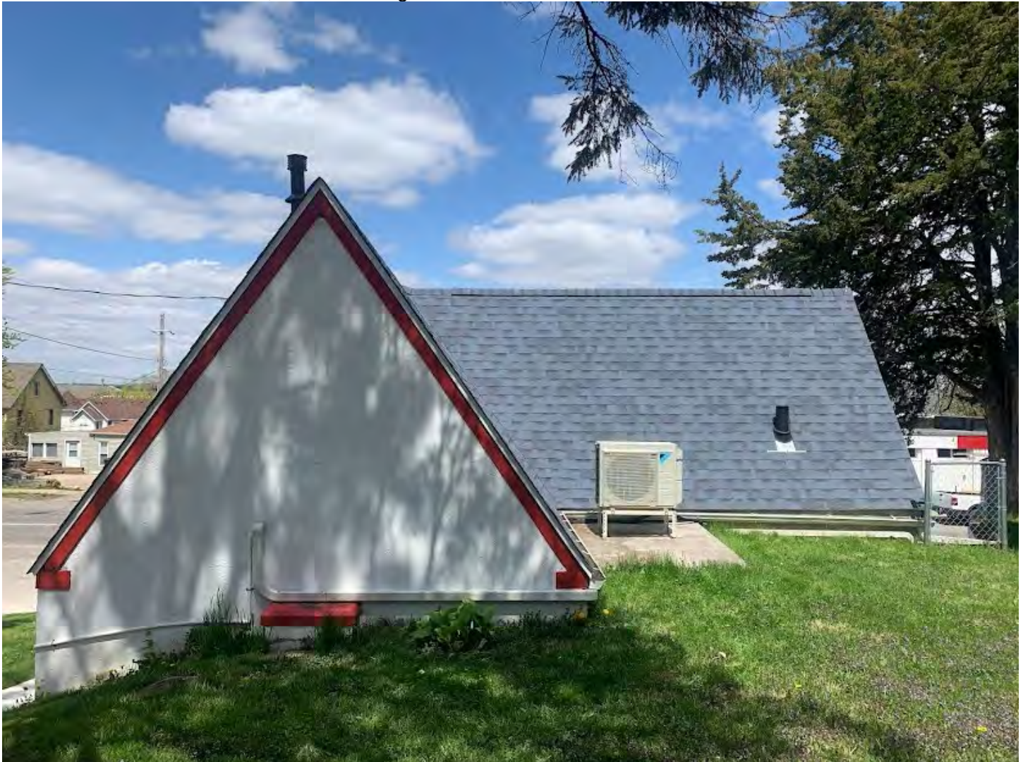
Photo 3 of 11: South facade, camera facing north.
