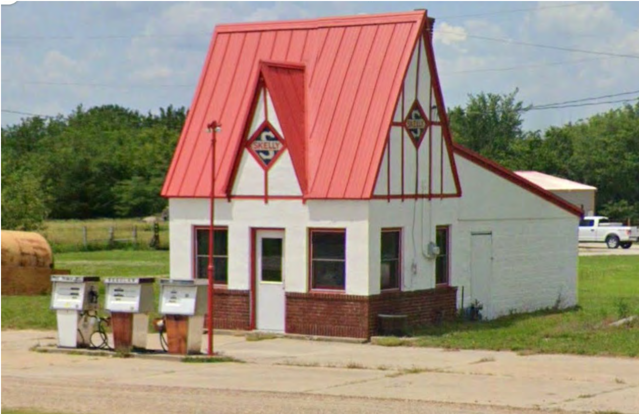
Figure 4. Skelly Service Station Cottage Type with rear addition (Lebo, Kansas).
