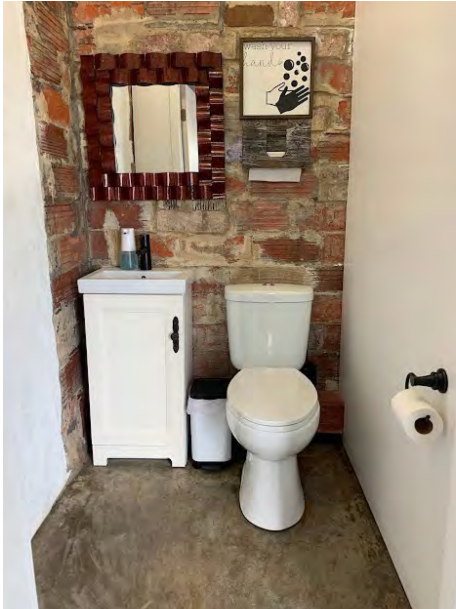
Photo 11 of 11: Constructed Restroom, camera facing southeast corner
