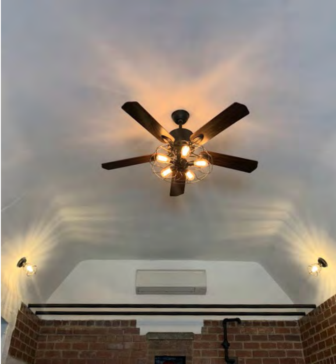
Photo 8 of 11: Service bay Ceiling repair, Original light fixture locations remain, camera facing south.
