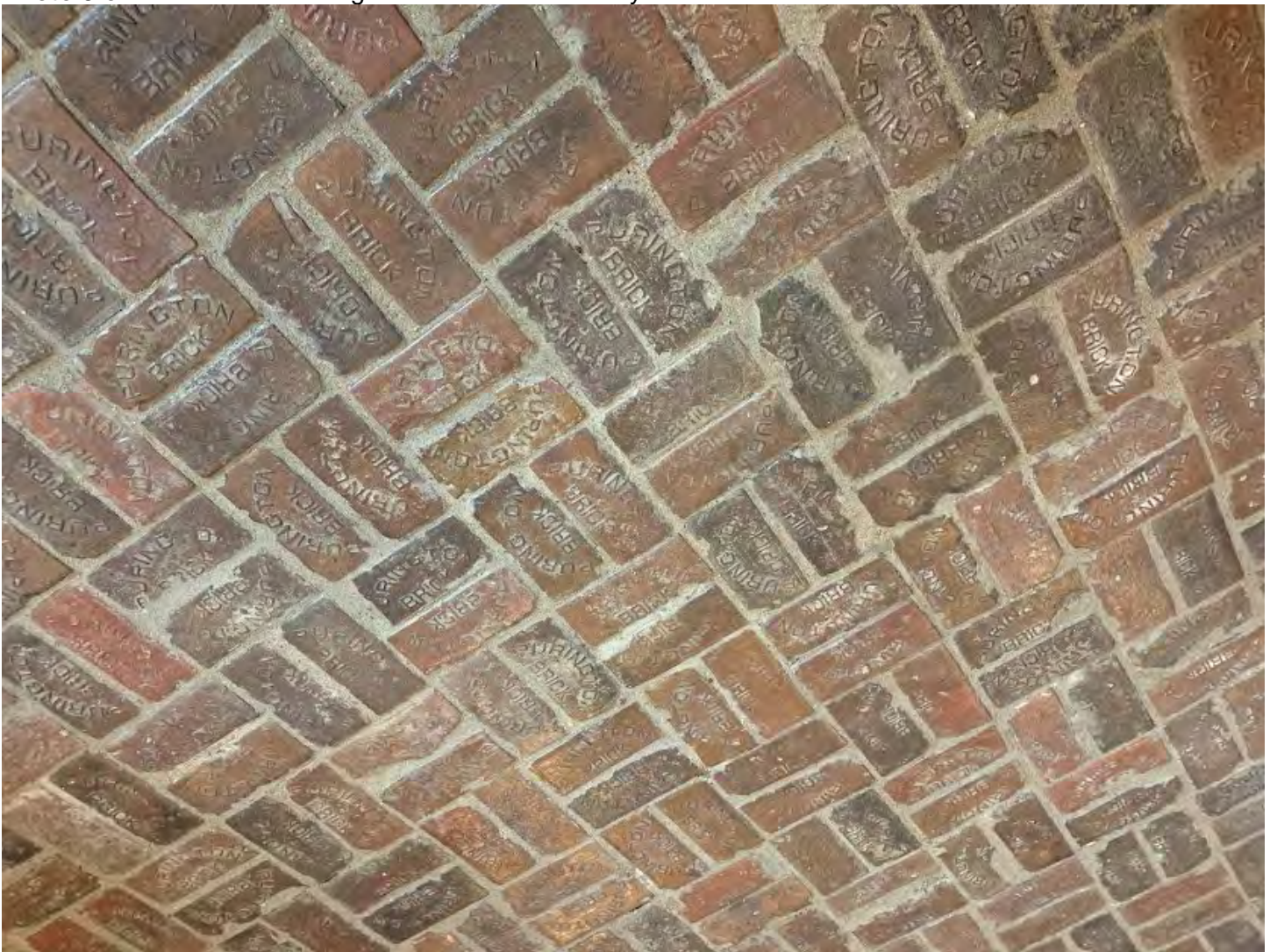
Photo 9 of 11: Restored Purington Bricks in service bay.
