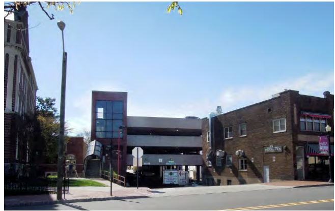
2.8-2: The North Fullerton Deck’s deep setback leaves it hard to find and foreboding. The Deck’s curb cut is too close to Bloomfield Avenue, resulting in a cramped approach and increased congestion.
