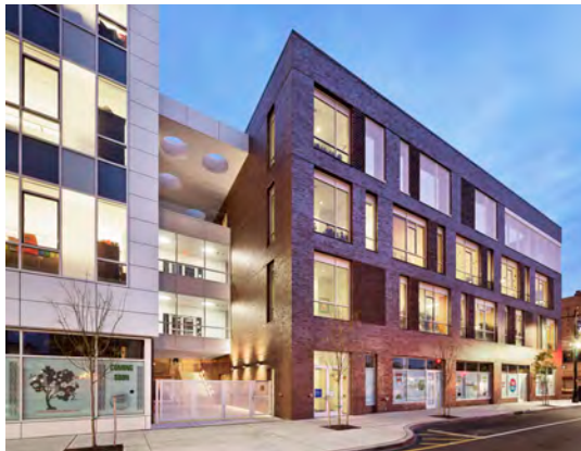
3.4-06: Historical material and style, such as brick and industrial openings, can be combined with new materials and expanded glazing to create a building suited for modern functions without seeming out of place in a walkable town center.
