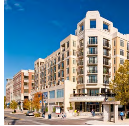
1.5-4: Encouraged: A prominent corner transition employs a deep entrance canopy and third-story stepbacks on the side to create a welcoming streetscape and an architectural rhythm easily legible to pedestrians.
