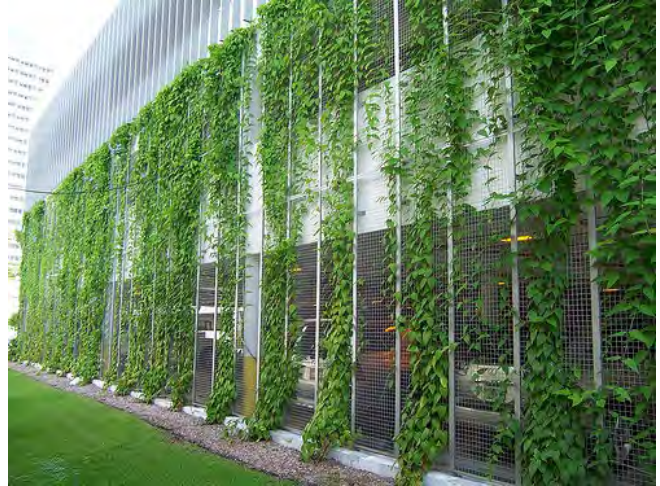
A planted green screen applied to a parking structure shades the interior, screens the deck structure, and visually softens the spaces around the deck.
