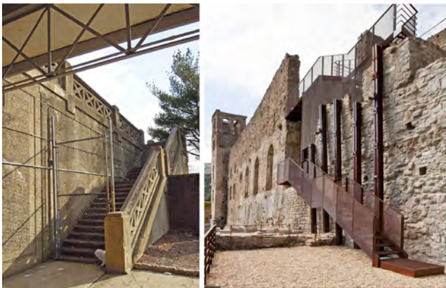
3.12-6: Existing but compromised historic elements, like the remaining Grove Street stair (above left), are excellent candidates for modern interventions that both restore function and dramatize old and new elements, as seen in a new steel stair providing access to a breach in the masonry of an ancient French fortification (above right).
