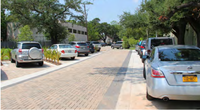
3.13-4: In this curbless parking area, sidewalk and street are one. Changes in paving material, texture, scale and color serve to designate different zones of use. In this paved landscape, pedestrian
