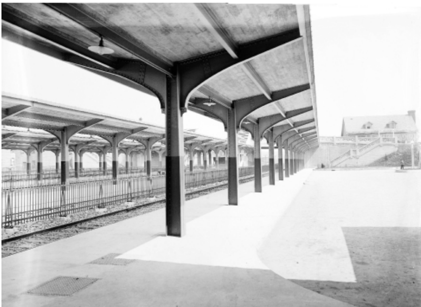
2.3-5: Looking east from the Waiting Room, c. 1915, the Platform Canopy closest to Bloomfield Avenue leads to a concrete stair (partly extant) that brought pedestrians up to the decorative concrete Grove Street bridge. The present-day brick wall facing Bloomfield Avenue (enclosing miscellaneous businesses, including Popeye's), was erected in the 1980's, immediately adjacent to the steel columns of this Canopy. The full concrete canopy remains intact and is visible inside, on the other side of the present-day brick wall.
