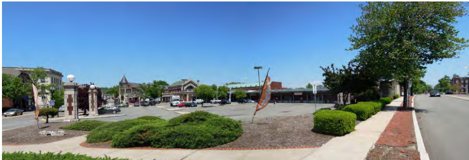
2.6-4: Looking west and north from the intersection of Bloomfield Avenue and Grove Street.
