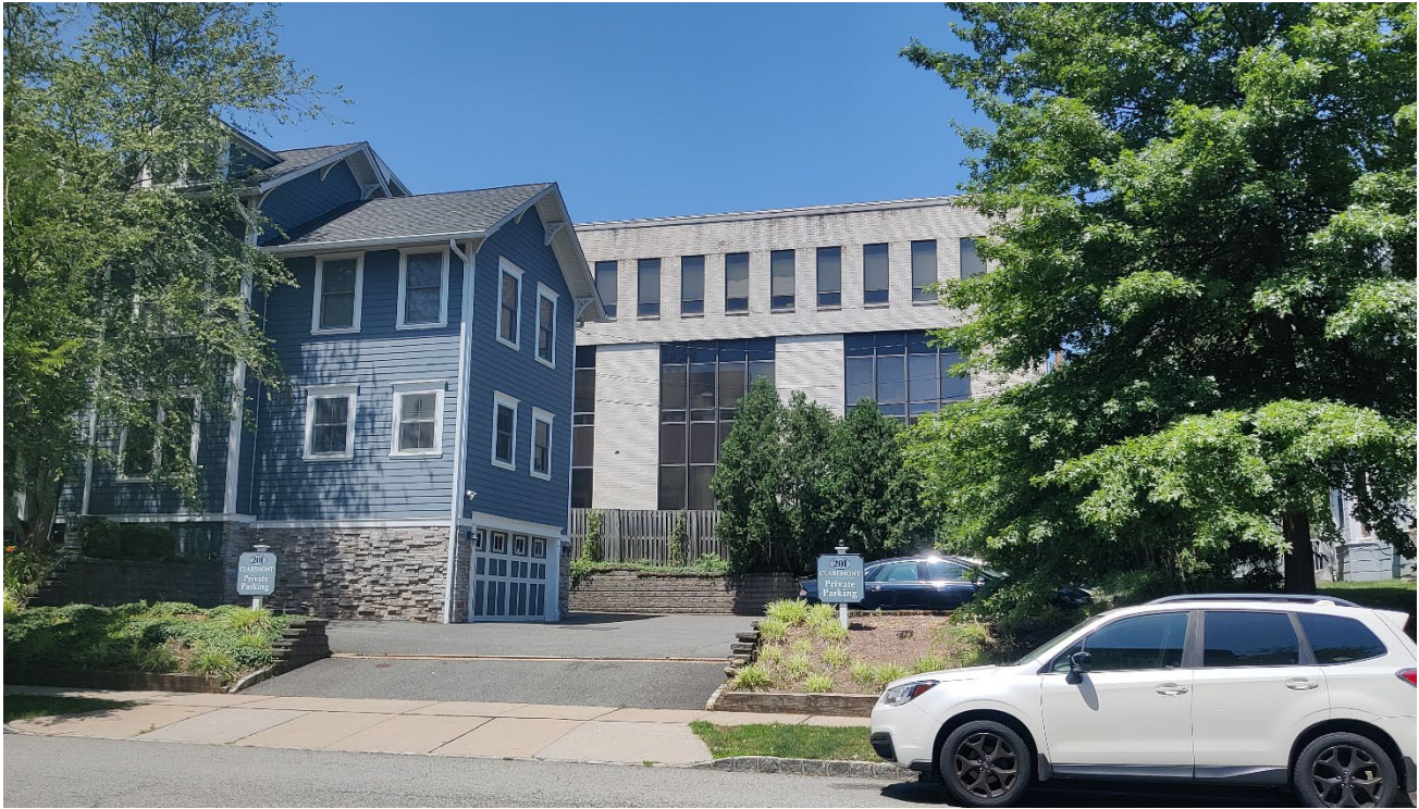
Figure 5: View of municipal building and office building at 201 Claremont Avenue looking west from North Fullerton Avenue.
