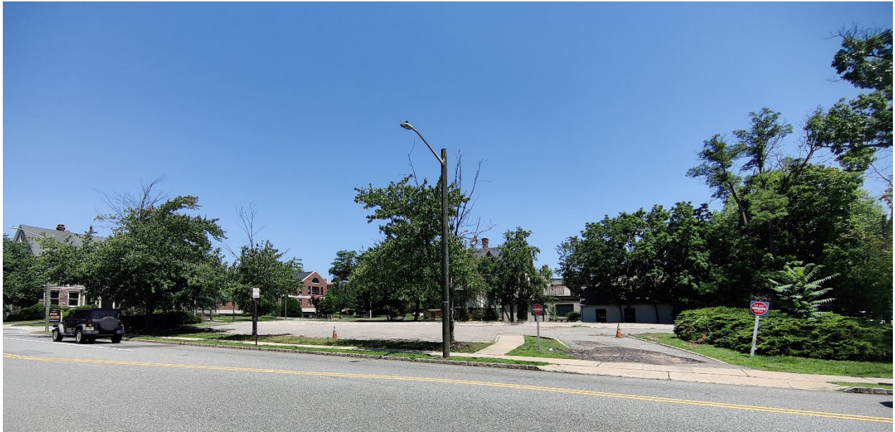
Figure 3: Photo of Lot 15 where the drive-through bank building has been demolished.
