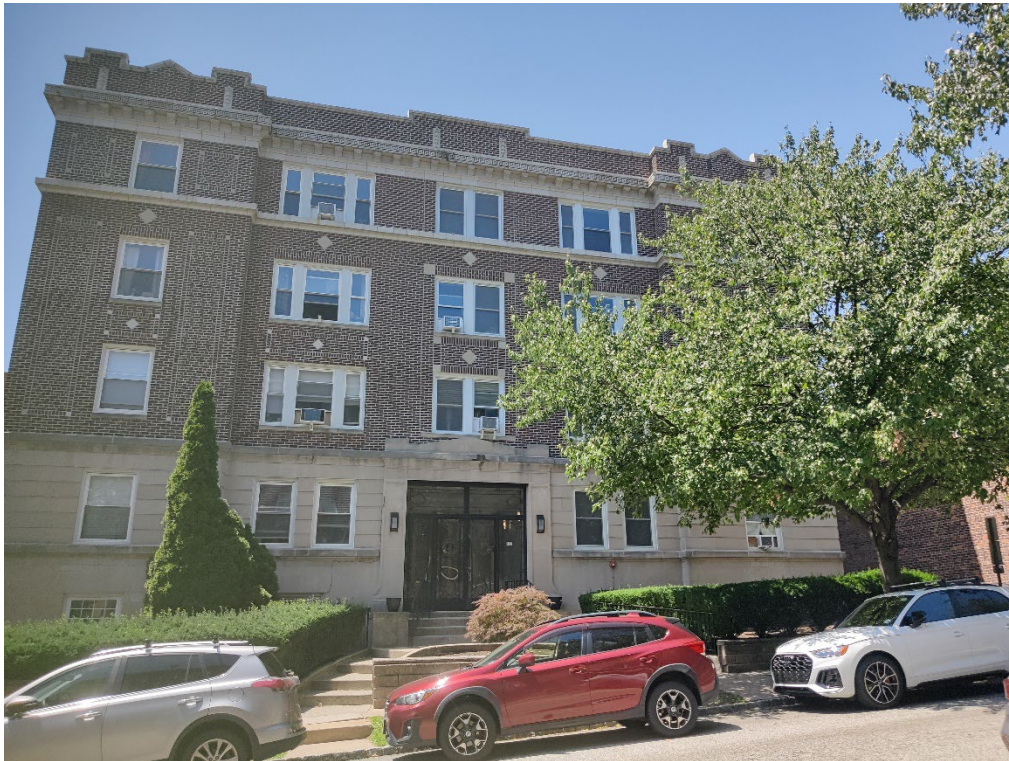
Figure 10: Four-story apartment building at 192 Claremont Avenue.
