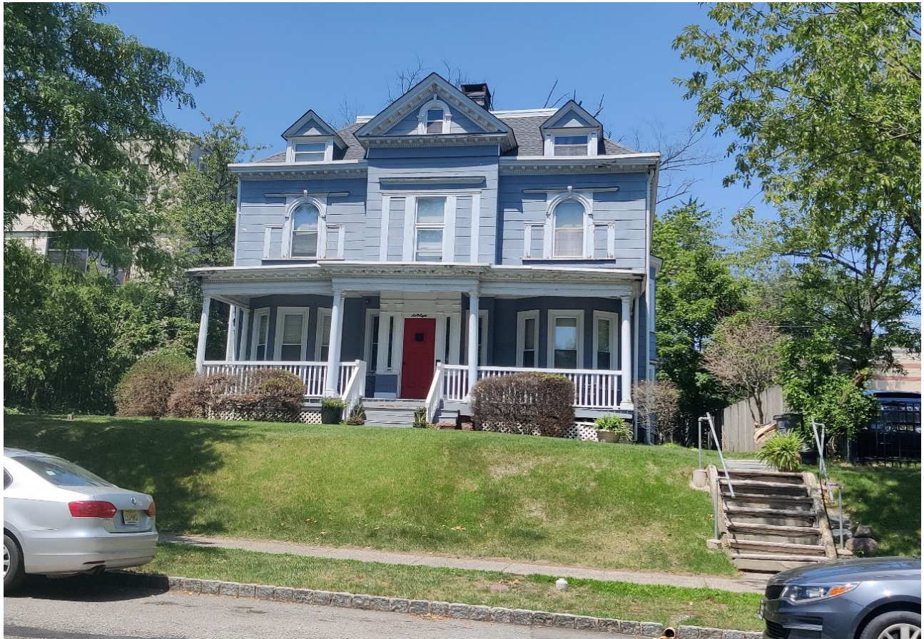
Figure 4: The Cornerstone House shelter located at 68 North Fullerton Avenue on Lot 12.
