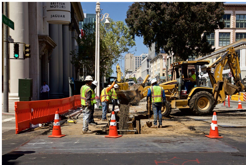
Figure 5.8 BRT Station Construction 16
