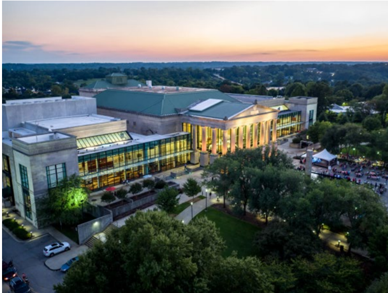
Figure 2.5 Martin Marietta Center for the Performing Arts 8
