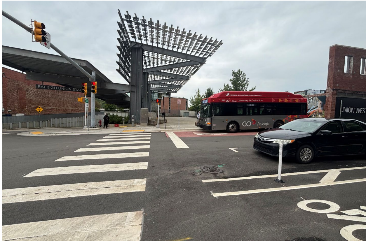
Figure 5.9 Raleigh Union Station with Intermodal Connections between Rail, Regional Bus, Local Bus, and Future BRT
