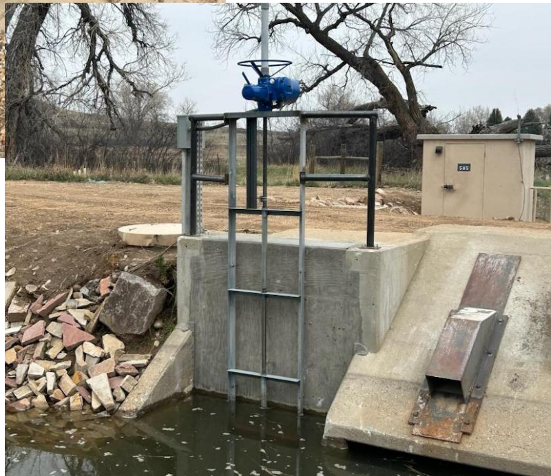
To the left, new turnout gates and actuators at the Holland Turnout. Below, is the turnout for Lefthand Creek.
