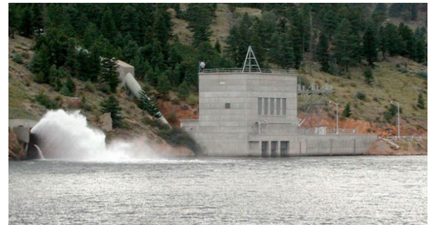
Mary's Lake Power Plant
