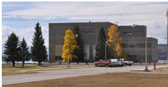
Farr Pump Plant
