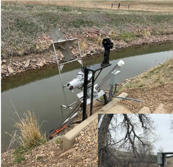
To the left, new turnout gates and actuators at the Holland Turnout. Below, is the turnout for Lefthand Creek.
