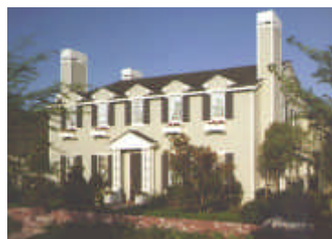
A strong roof punctuated by a row of dormers with windows
