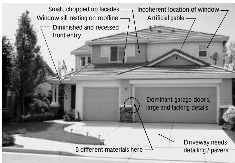
Elements that detract from the architecture quality
