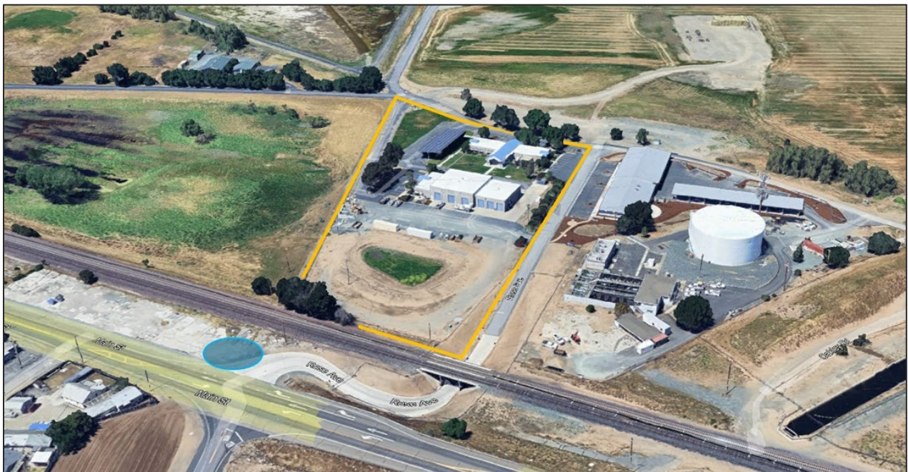
Figure 1 – Project Site (General sign location in blue circle, ISD facility outlined in orange)
