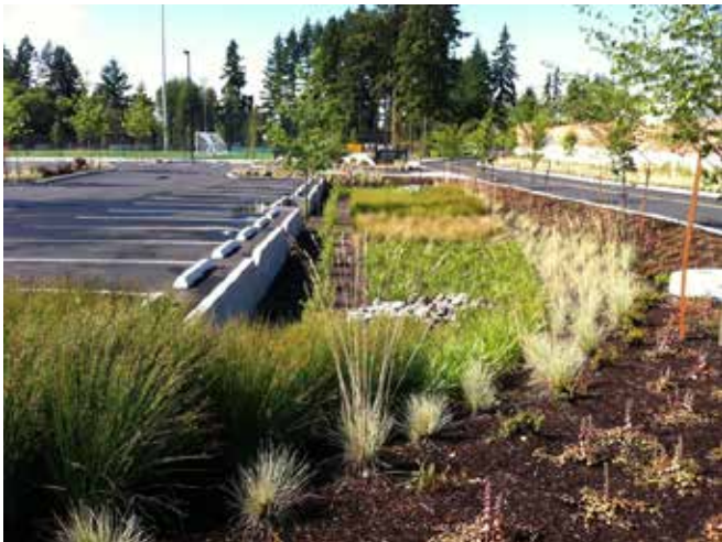
Incorporate Bioswales to Maximize Stormwater Infiltration
