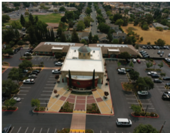
F. Civic Center Roof Replacement Project
