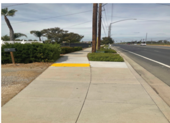
E. Curb, Gutter, & Sidewalk Repair Project
