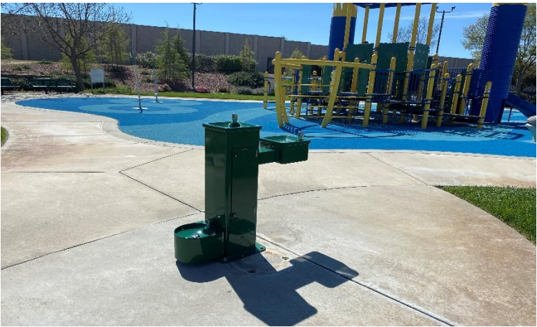
P. City Parks Drinking Fountain Replacement Project
