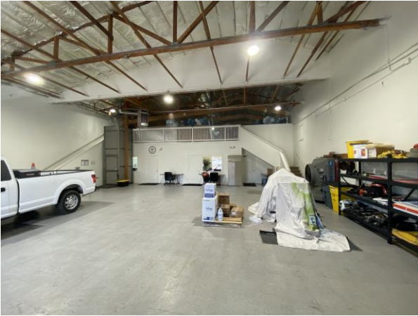
M. Public Works Operations Building Remodeling Project
