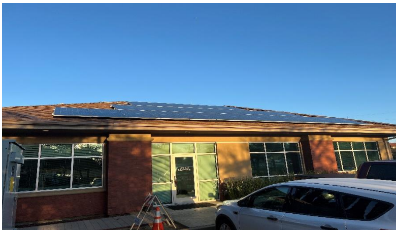
H. City Hall Rooftop Solar Power Project
