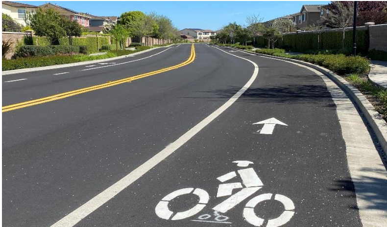
G. FY 2022/23 Street Repair and Resurfacing Project
