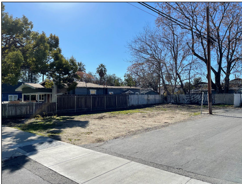
Project Site – View looking southwest
