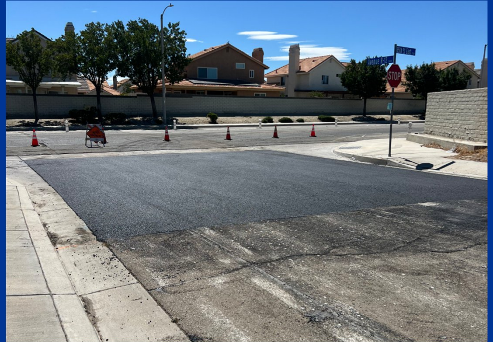
PN 904 Mill and Overlay at Intersection Stop Point
