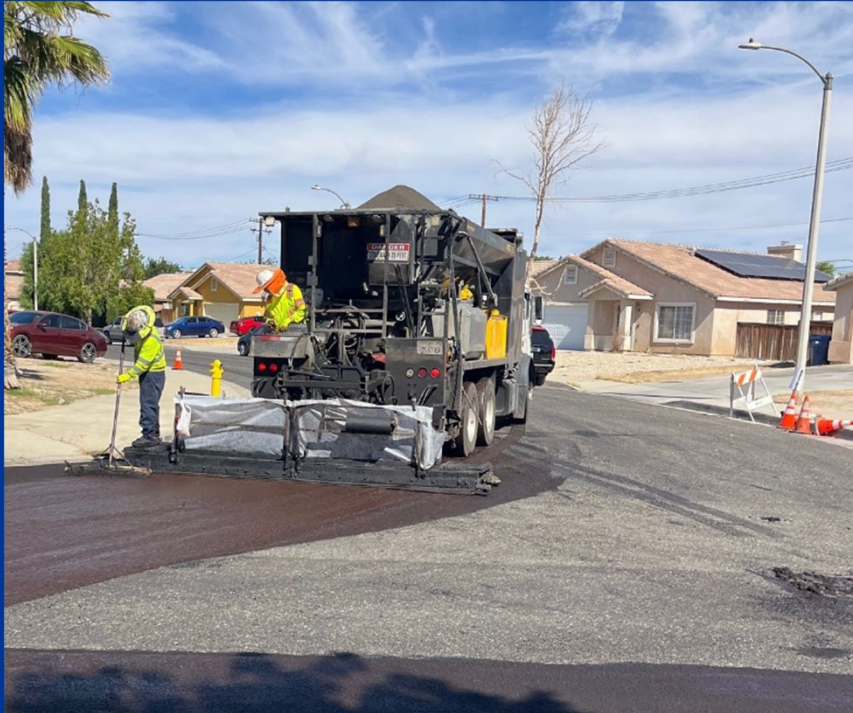
PN 904 Slurry Seal Placement over ARAM Chip Seal
