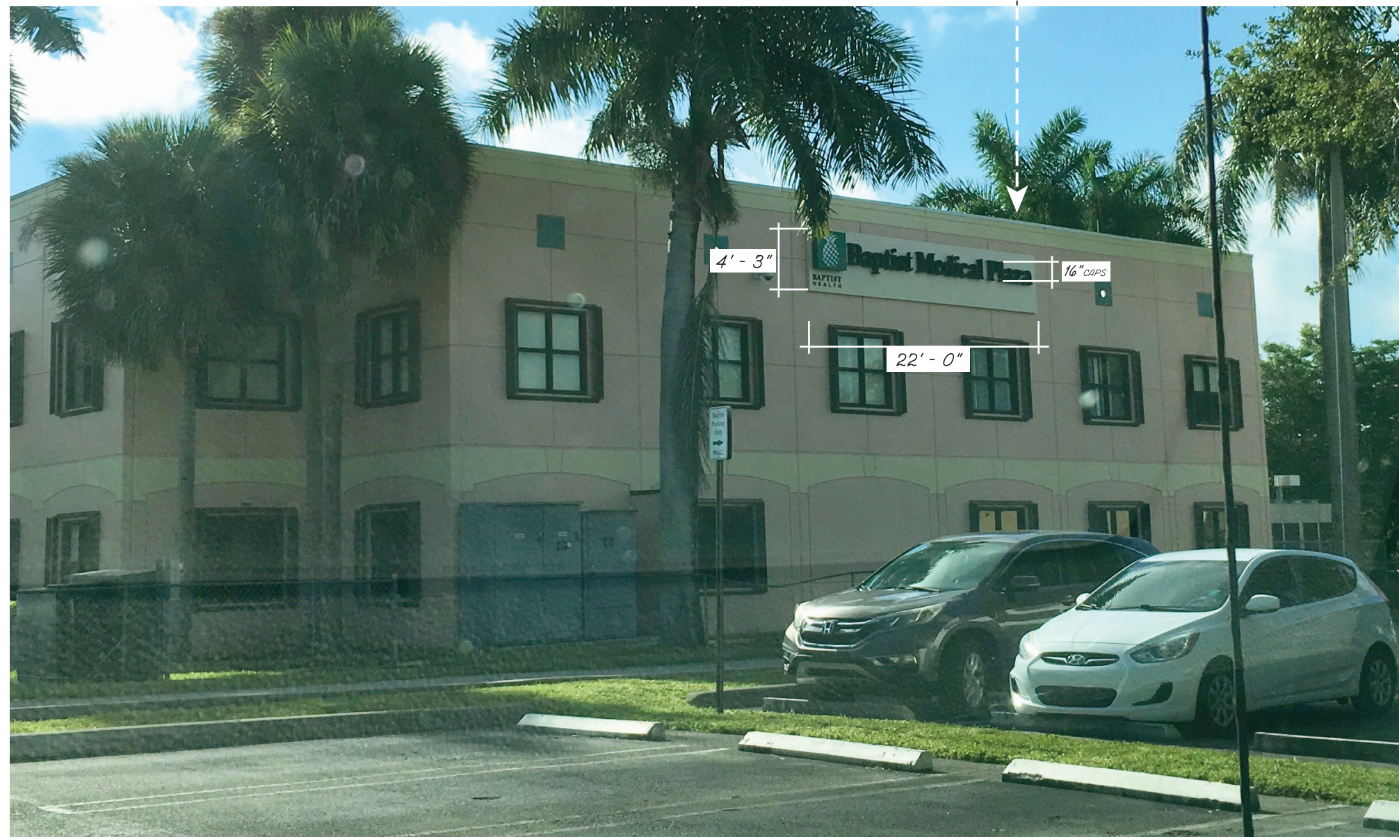
PHOTO OF EXISTING WEST FACADE
