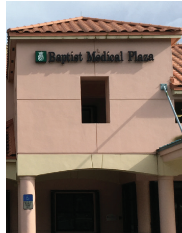
North Facade (16.6 s.f.)
