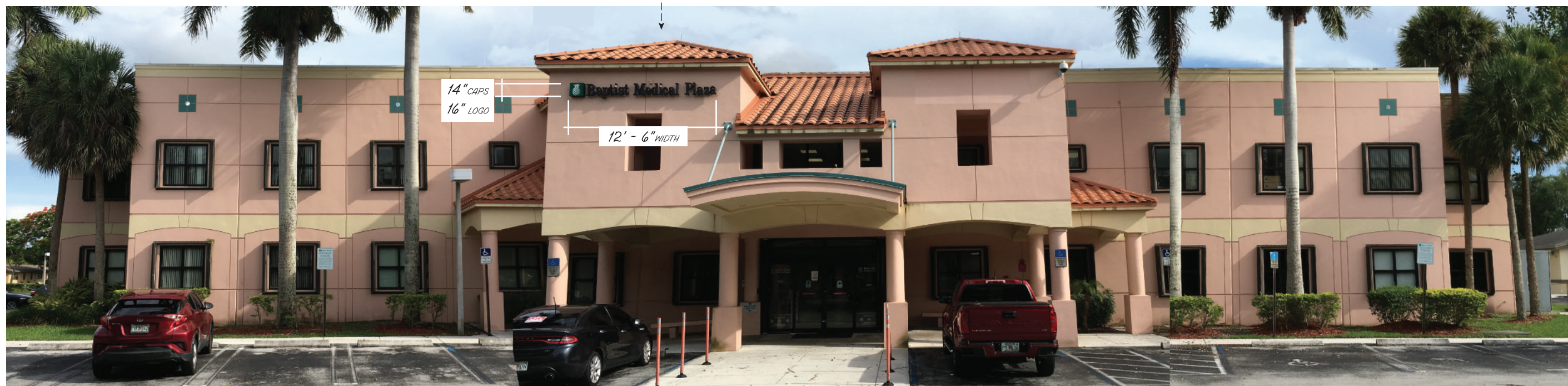
PHOTO OF EXISTING NORTH FACADE
