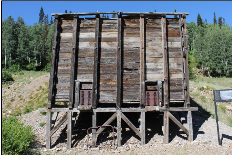
Figure 69. Overview of Little Bell Mine Ore Bin, facing west. Note deteriorated boards at top of walls.
