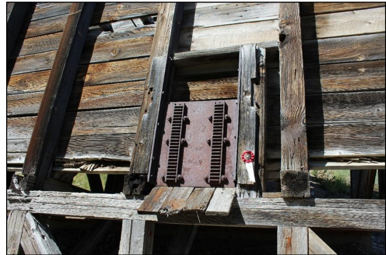
Figure 72. Close up of north gate for Little Bell Mine Ore Bin, with damaged and missing boards visible, facing west.
