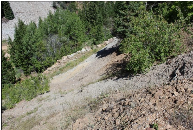
Figure 21. Overview of American Flag Mine Waste Dump slope, facing north. Note areas of vegetation cover mixed with areas of unvegetated tailings.
