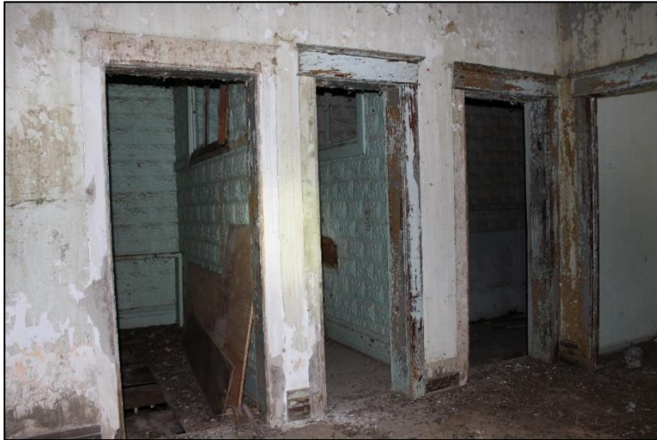
Figure 11. Interior of Judge Mining and Smelting Company Office, first floor, facing south-southwest. Note the use of pressed tin for wall finishes.
