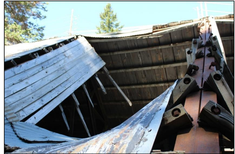
Figure 10. Detail of collapsed roof with twisted wood purlins visible in foreground at right, facing west-northwest.
