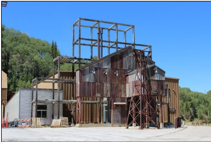
Figure 25. Overview of Ontario Mine Shaft No. 3 building north of hoist, facing north. Note square-set timbering and tram tower, later additions to building.
