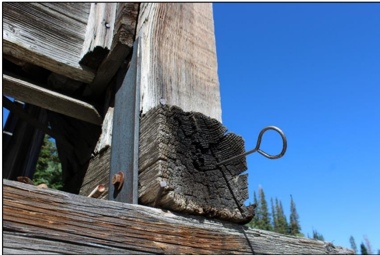
Figure 71. Deteriorated structural member, north end of Little Bell Mine Ore Bin, facing northwest. Note the 1-foot-long probe illustrating depth of rot.
