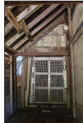
Figure 16. Entrance to Anchor (Daly-Judge) Drain Tunnel, facing southwest. Note modern metal posts supporting roof and modern gate over entrance.
