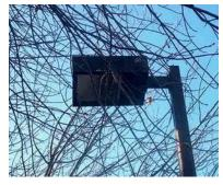
upper lot are actually above the trees, as shown in the photo to the right, which means that little light actually gets down to the path. It may be desirable to provide new lighting. This lighting could have a closer spacing between lights with shorter pole lengths, which would keep the light below the trees. These new lights could be in the same historic style as those currently in use in the Sandridge Lots, as shown in the photo to the left.
