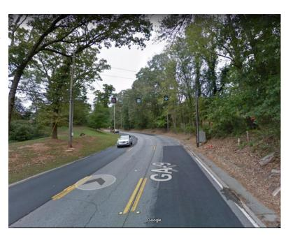
Some outcomes of this reversible lane deployment have been a higher collision rate along the reversible lane section of SR-9. There is a lot of horizontal curvature, and it was found that collision rates were higher than for similar facilities without reversible lanes.
