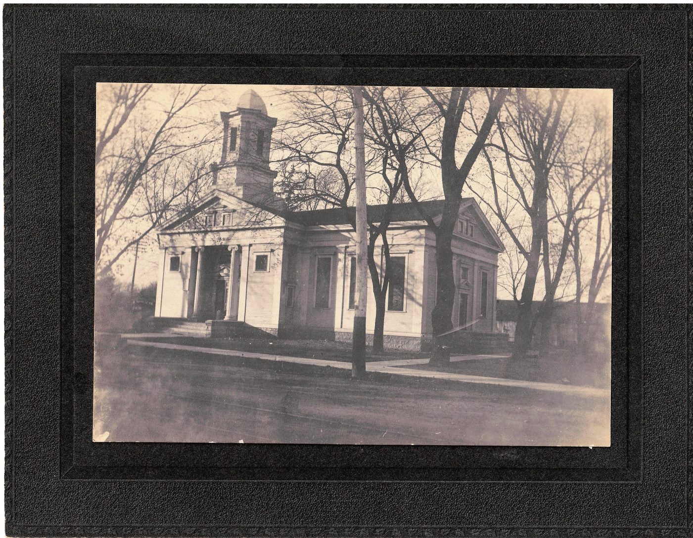
South Facade following the 1906 Construction
