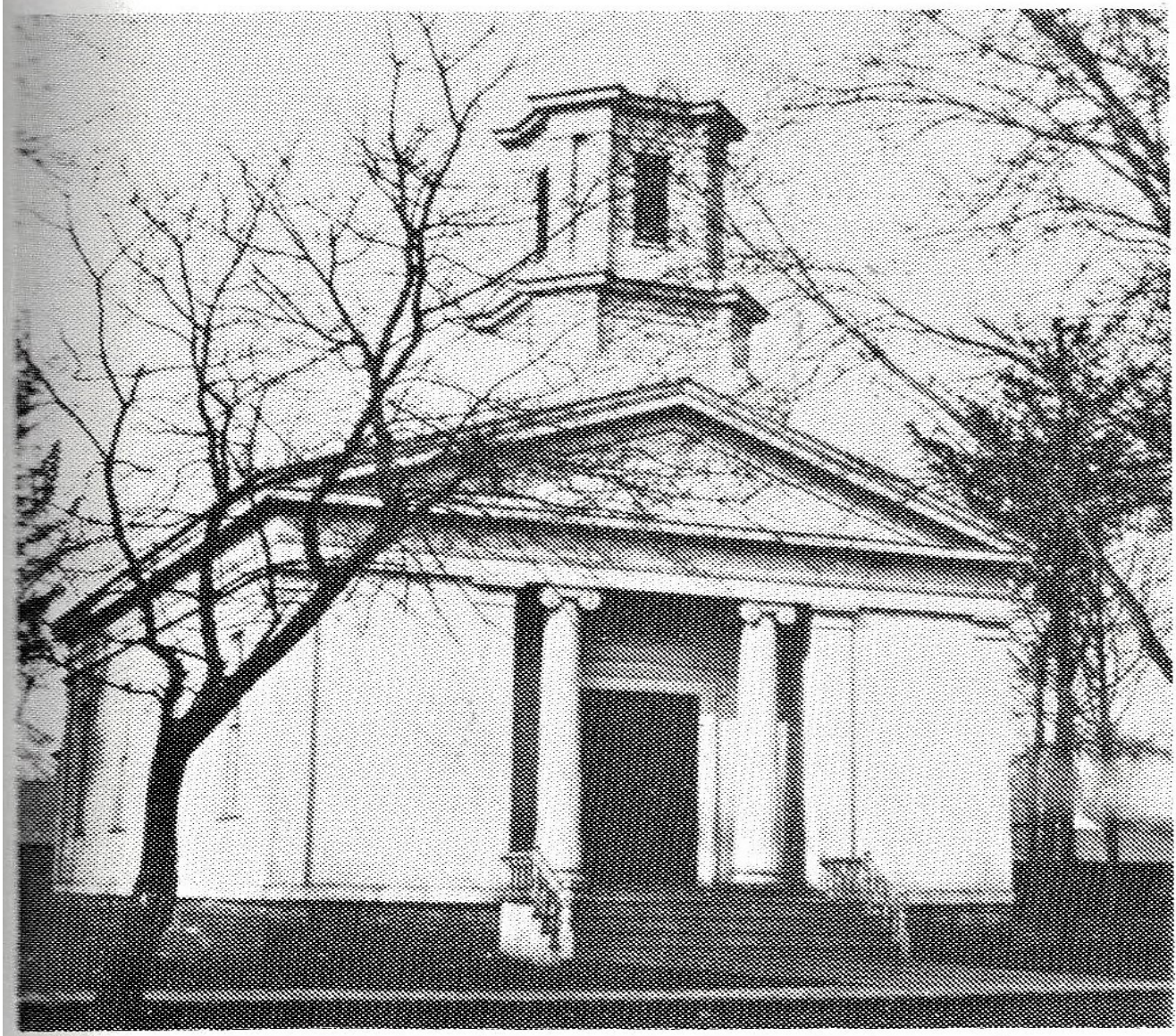
South Facade following the 1850 Construction
