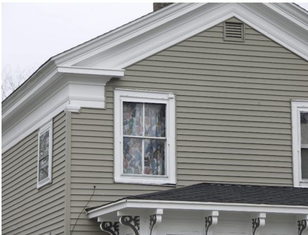
Detail, gable front Camera facing northeast
