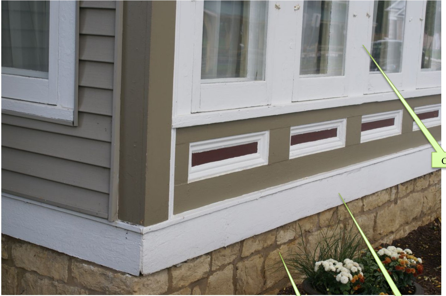
Plate 5 – Corner detail at siding and foundation
