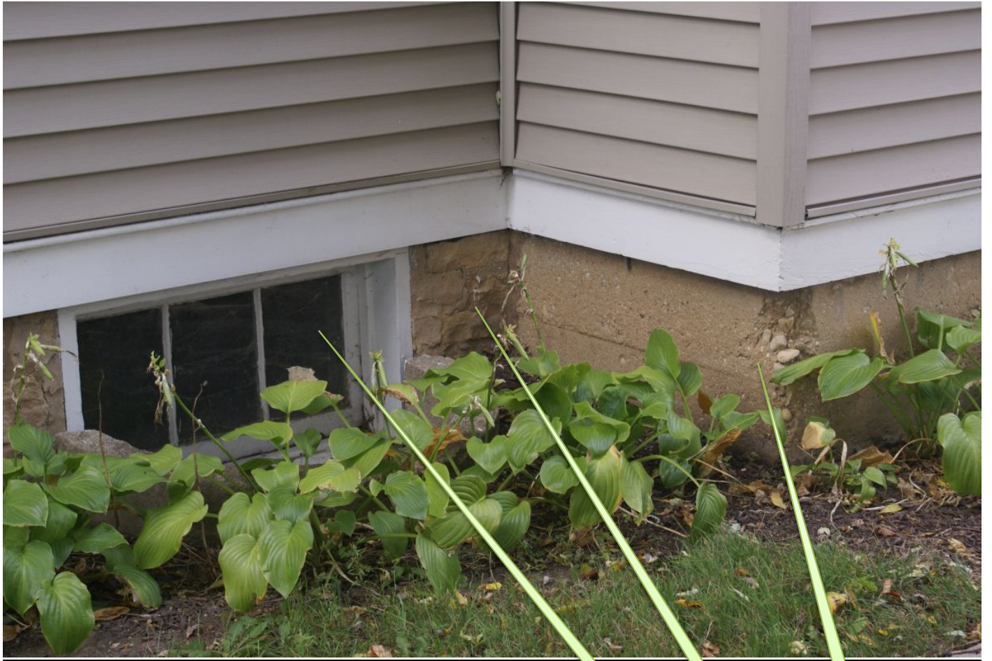
Plate 12 – Foundation wall detail – original with addition photo credit: Leif Hendricksen
