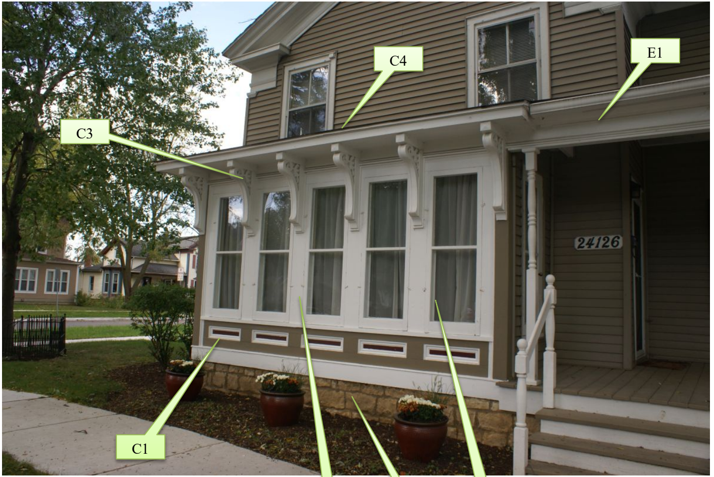
Plate 2 – South façade two-story portion photo credit: Leif Hendricksen
