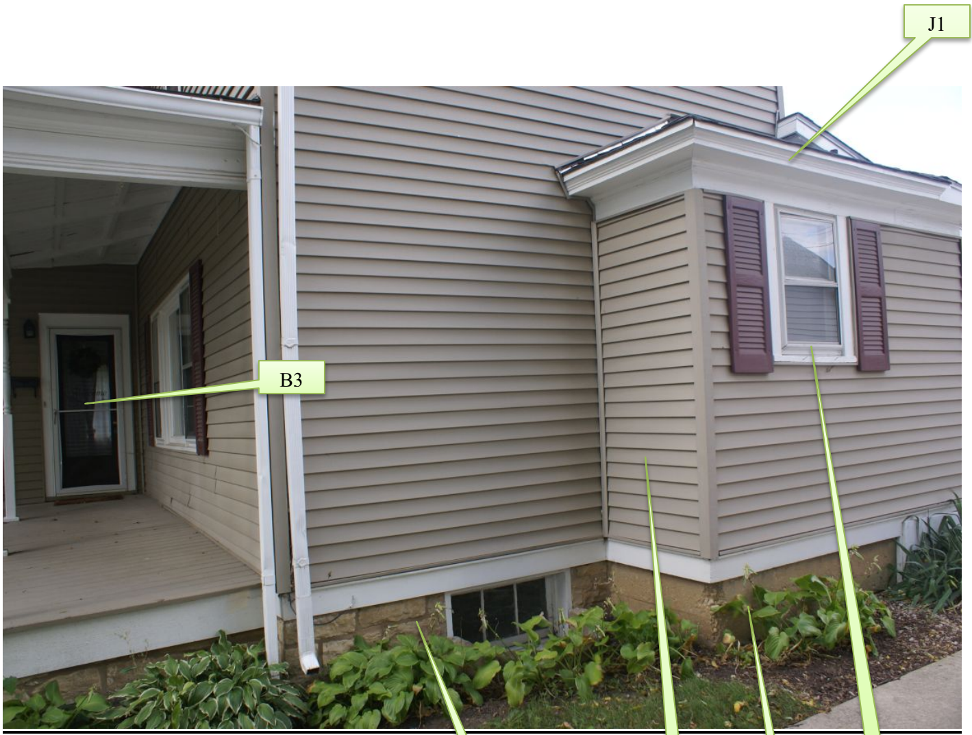
Plate 11 – East façade with single-story addition photo credit: Leif Hendricksen
