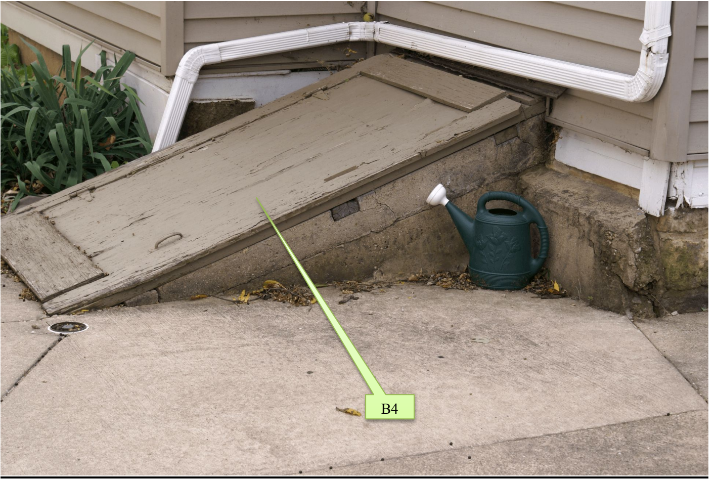
Plate 15 – Basement access photo credit: Leif Hendricksen
