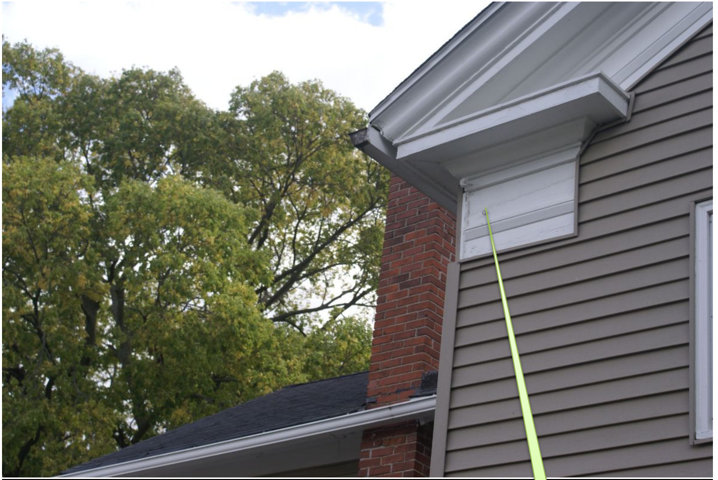
Plate 9 – Roof overhang, eave and fascia detail photo credit: Leif Hendricksen
