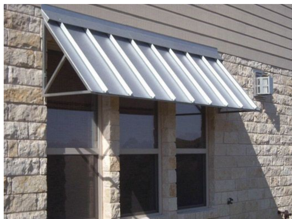
CUSTOM STANDING SEAM METAL AWNING
