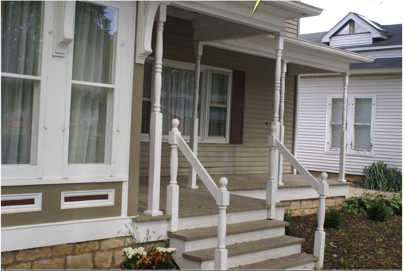
Plate 4 – South façade detail at porch
