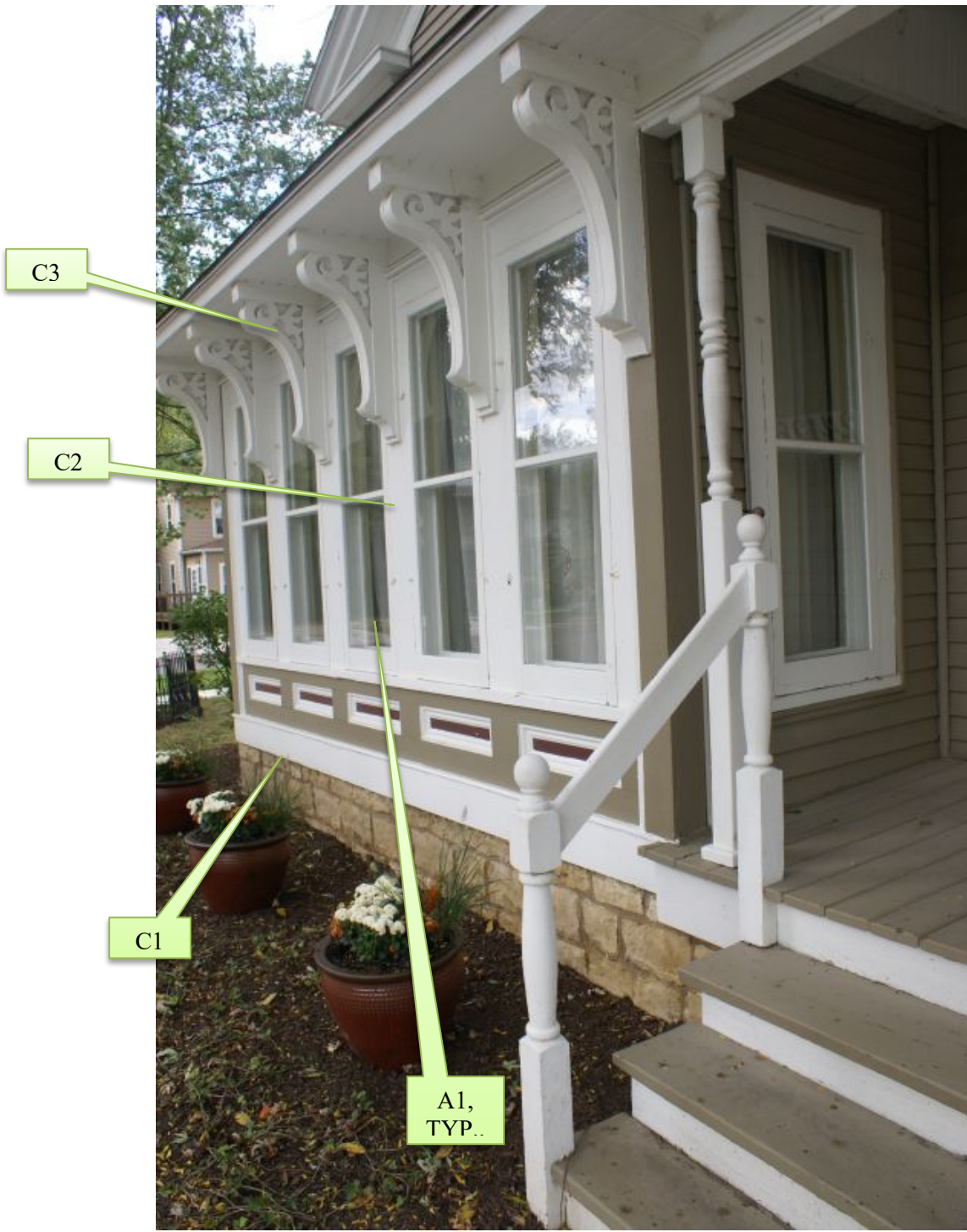
Plate 3 – South façade detail at windows photo credit: Leif Hendricksen
