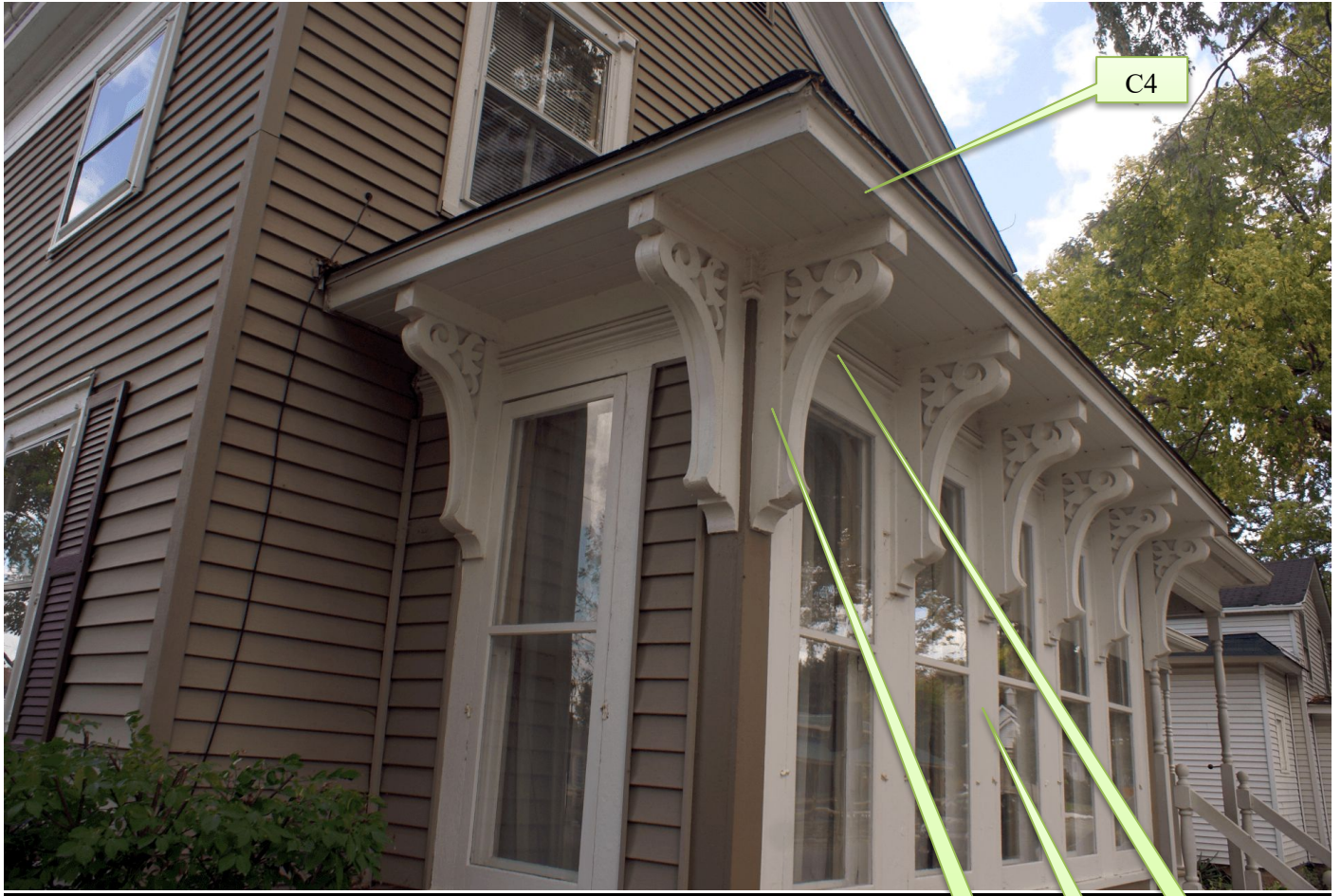
Plate 13 – Southwest corner façade at single-story portion photo credit: Leif Hendricksen
