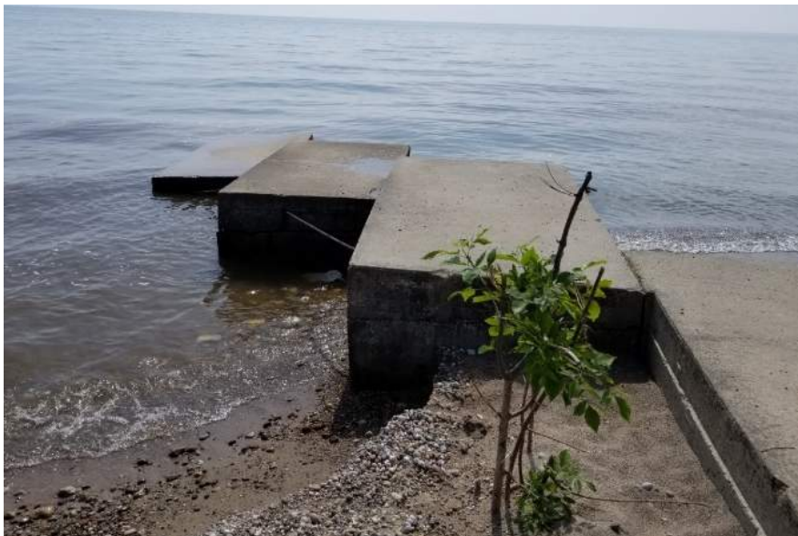
Figure 4: Tobin Creek Discharge and Groin Looking East
