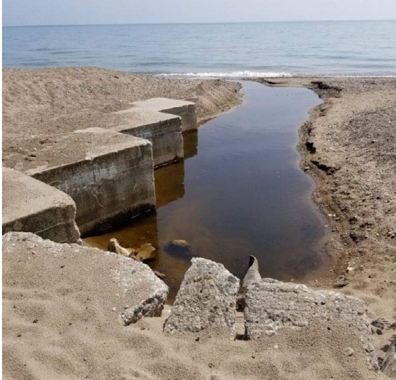
Figure 7: Local Drainage Discharge Looking East
