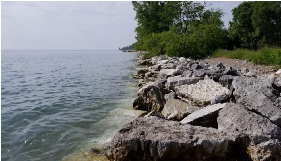
Figure 2: Existing Revetment Looking South
