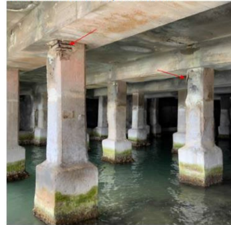
Pile V, Row 1 with exposed rebar.
