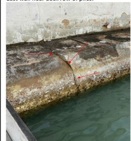
Footing at Bent 0
