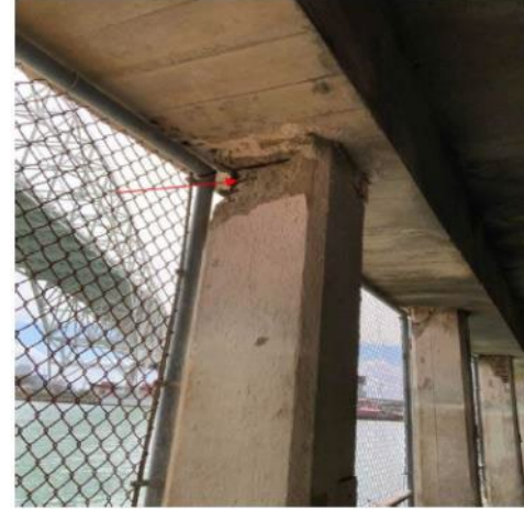
Pile V, Row 1 with exposed rebar.
