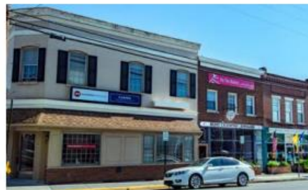
Figure 147. Main Street Businesses with traditional storefront architecture.
