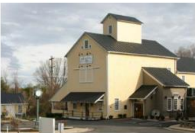
Figure 146. The landmark architecture of the Magnolia Mill.
