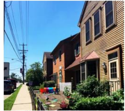
Figure 152. Example of commercial frontage that has lower level parking and entries to the rear
