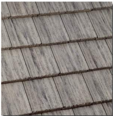
Roof: Ponderosa - 5511 Flintridge Gray Mfr: Eagle Roofing
