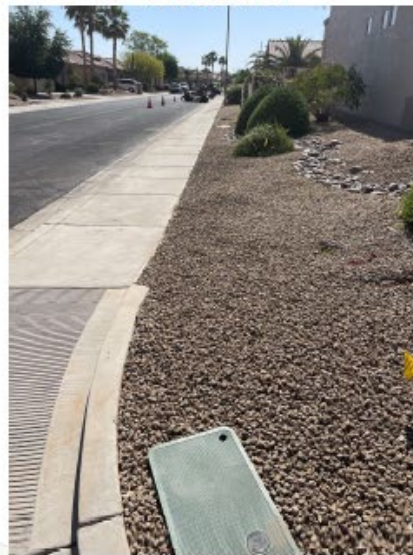
Completed HH At the edge Marks cleaned
