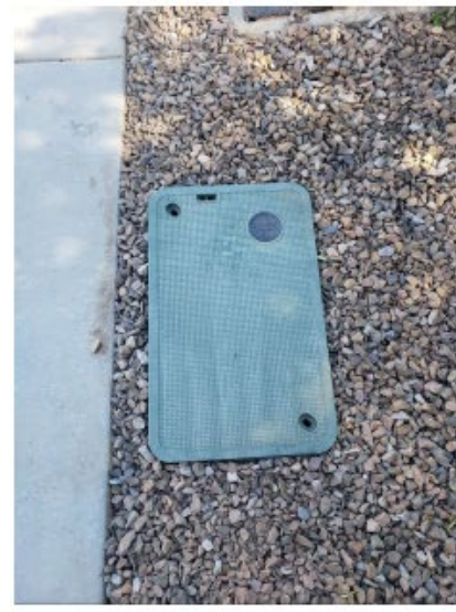
Completed HH Along ROW
