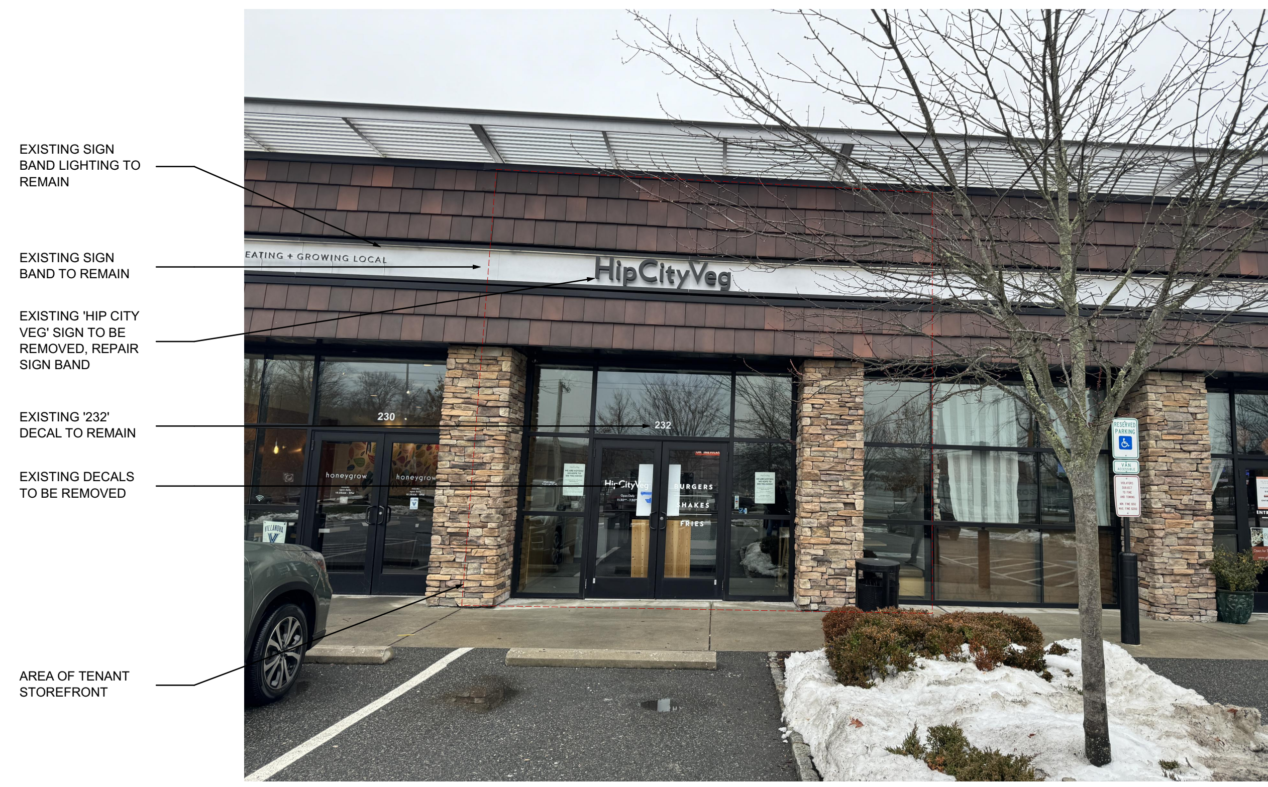
3 EXISTING CONDITIONS PHOTO SCALE: 1:7.43
