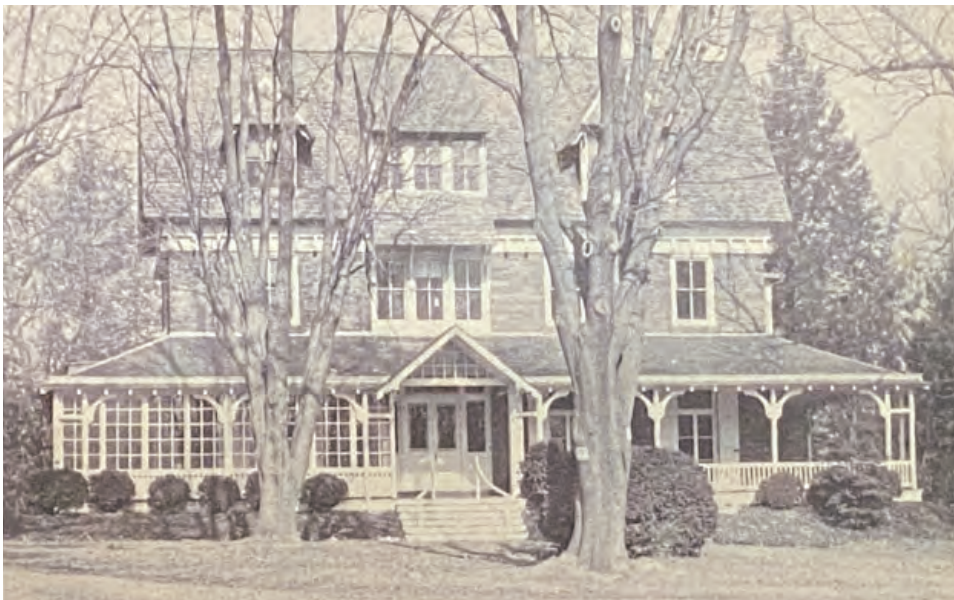
ILLUSTRATION 2 PHOTO OF SOUTH FACADE, DATE UNKNOWN
